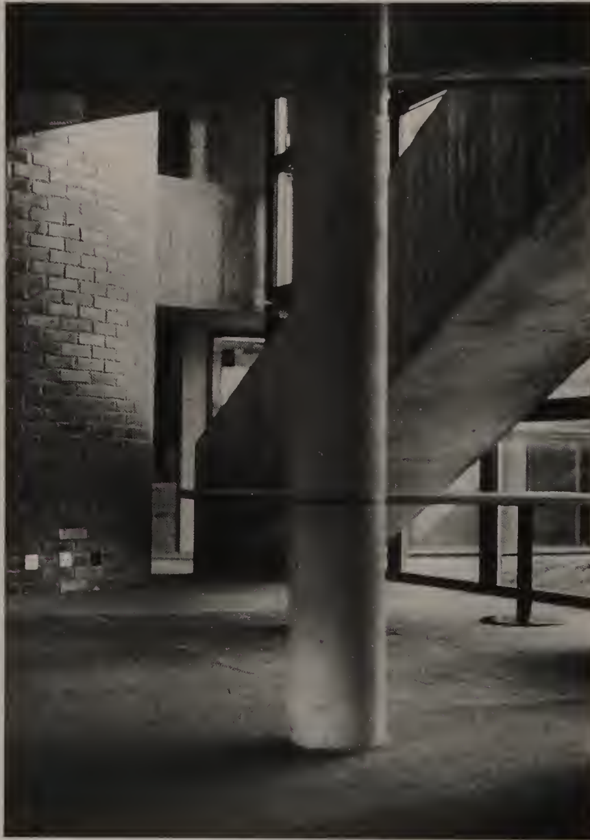
Concrete column, Skådalen School for Deaf Children. Oslo, Norway. 1972.
