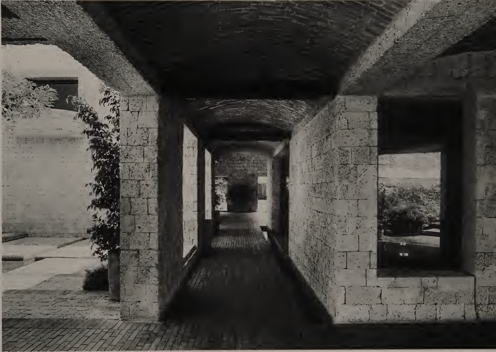
Guest House. Passage between Library and Patio del Roble Morado.
