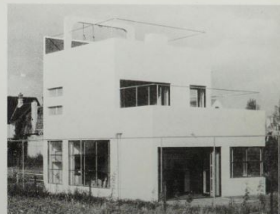
Above Modern Movement architects prided themselves on designing houses that were tailored to the needs of modern living. The Caneel House in Brussels, designed by J. H. De Koninck in 1931, had two roof terraces, one of which was fitted out as an open-air gymnasium. This feature reflects the importance attached to sunbathing and outdoor exercise at this date.
