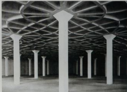
Right Pier Luigi Nervi combined the talents of the engineer with the creativity of the artist: the pattern of the strengthened radiating ribs moulded into the concrete ceiling in his Gatti Wool Factory in Rome of 1951-3 follow the sinuatic lines of stress calculated for this structure.
