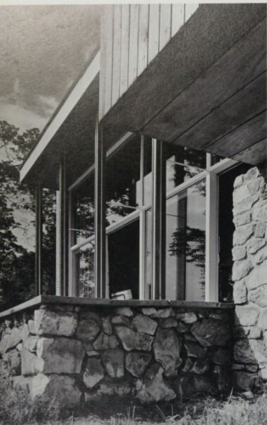
Expressive and varied surface textures were a distinctive feature of 1950s architecture. Above Peter Womersley's Farley Hey in West Yorkshire, dating from 1953, combines rough stonework with tongue-and-groove wooden cladding on the outside.
