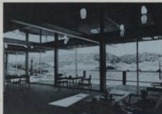
Above The Shulman House, Laurel Canyon, Los Angeles, designed by Raphael Soriano in 1950, seen here under construction. This house, built for the photographer Julius Shulman, is composed of two distinct blocks. On the left is the studio and on the right is the main house; the two are connected by a covered walkway. The modular steel-framed post-and-beam construction method is clearly visible here. Right An advertisement for the Bethlehem Steel Company promoting steel-frame construction for 'Contemporary' houses.
