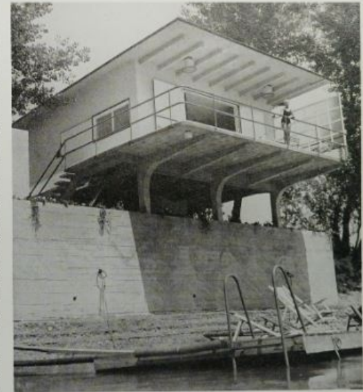
Above House on the Danube in Hungary designed by Ludwig Mies van der Rohe in 1928. Not only was the structural framework of this house constructed using reinforced concrete, but the floors and the roof were as well. In places, the concrete was left exposed, revealing the impress of the shutters used to contain it while it was being poured.
