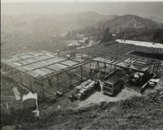
Above The Shulman House, Laurel Canyon, Los Angeles, designed by Raphael Soriano in 1950, seen here under construction. This house, built for the photographer Julius Shulman, is composed of two distinct blocks. On the left is the studio and on the right is the main house; the two are connected by a covered walkway. The modular steel-framed post-and-beam construction method is clearly visible here. Right An advertisement for the Bethlehem Steel Company promoting steel-frame construction for 'Contemporary' houses.
