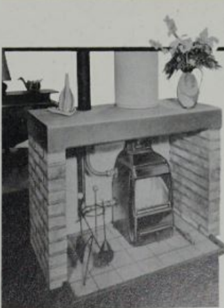
Above Discreet or hidden heating systems were favoured during the 1950s. One example of a new system which came on the market at this time was the slimline Wallstrip radiator produced by Copperad which ran round the room at skirting board level. Left: The Parkway connector fire, which could burn smokeless fuel, was selected by the architect Basil Spence in 1958 for new housing built at Bealton New Town. Note the 'Contemporary' style ball-and-spoke accessories in the hearth and the use of the fireplace as a room divider.
