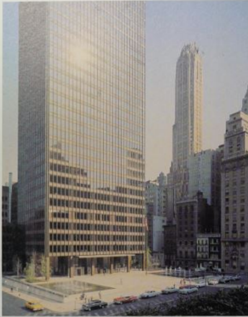
One of the great achievements of Modern Movement architecture was to increase the amount of natural light in buildings. Above: The Seagram Building in New York, designed by Mies van der Rohe in 1958, demonstrates the concept of curtain wall window systems as applied to a tall office block. Here, glass is used as the main cladding material in place of masonry.
