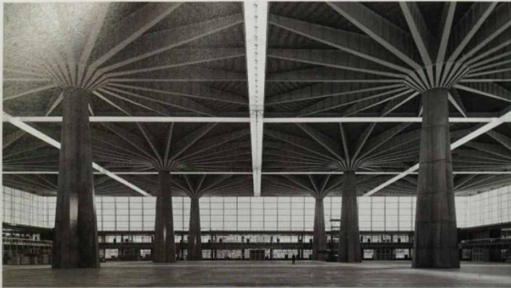
Pier Luigi Nervi was the most talented structural engineer of his age. His achievements using reinforced concrete, or 'ferro-cemento' as he called his particular version of this material, are still unrivalled today. Above: The Palazzo del Lavoro at Turin, dating from 1961, combines massive concrete columns with exposed radiating steel girders. Even when moving away from total reliance on his favoured material, concrete, Nervi produces a startling and original design. Right: Detail of the angular concrete pilasters supporting the dome of the Palazzo dello Sport, the larger of Nervi's two Olympic 'sports palaces', designed in collaboration
