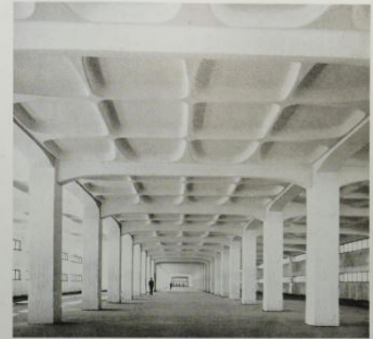
Building with concrete was seen as an heroic enterprise during the 1950s. Top Interior of Tobacco Factory at Bologna designed by Pier Luigi Nervi in 1951-2. The reinforced concrete ceiling was created in large sections in situ by pouring concrete from above onto re-usable 'ferrocemento' formers raised on scaffolding.
