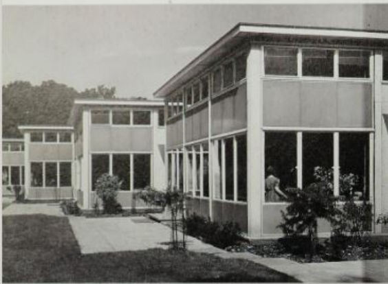
Above: Templewood School, Welwyn Garden City, designed by Hertfordshire County Council Architects Department under C H Ashin, built on a modular system using an 8'1/2" x 2.5m grid and standardized prefabricated components. As a result of the adoption of this modular system of building, a total of one hundred schools were built in the county of Hertfordshire alone between 1946 and 1955.
