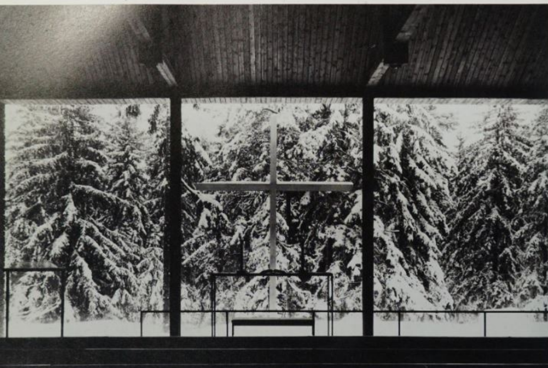
Above Chapel at Otanemi Technical University in Finland designed by the husband-and-wife team of Kaija and Heikki Siren, built during 1956-7. The installation of a glass curtain wall at the end of the church, so that the trees behind form the backdrop to the altar,
