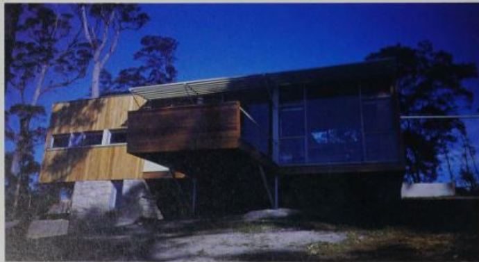
Above Particularly sympathetic was the use of re-stained cladding on many of Richard Neutra's houses, such as the Trowick House. Right Cedar boarding exported from countries such as Canada was widely used for exterior cladding during the 1950s. Here, it is shown applied as the facing material to a house at Kurrajong Heights near Sydney, Australia, designed by Harry Seidler.
