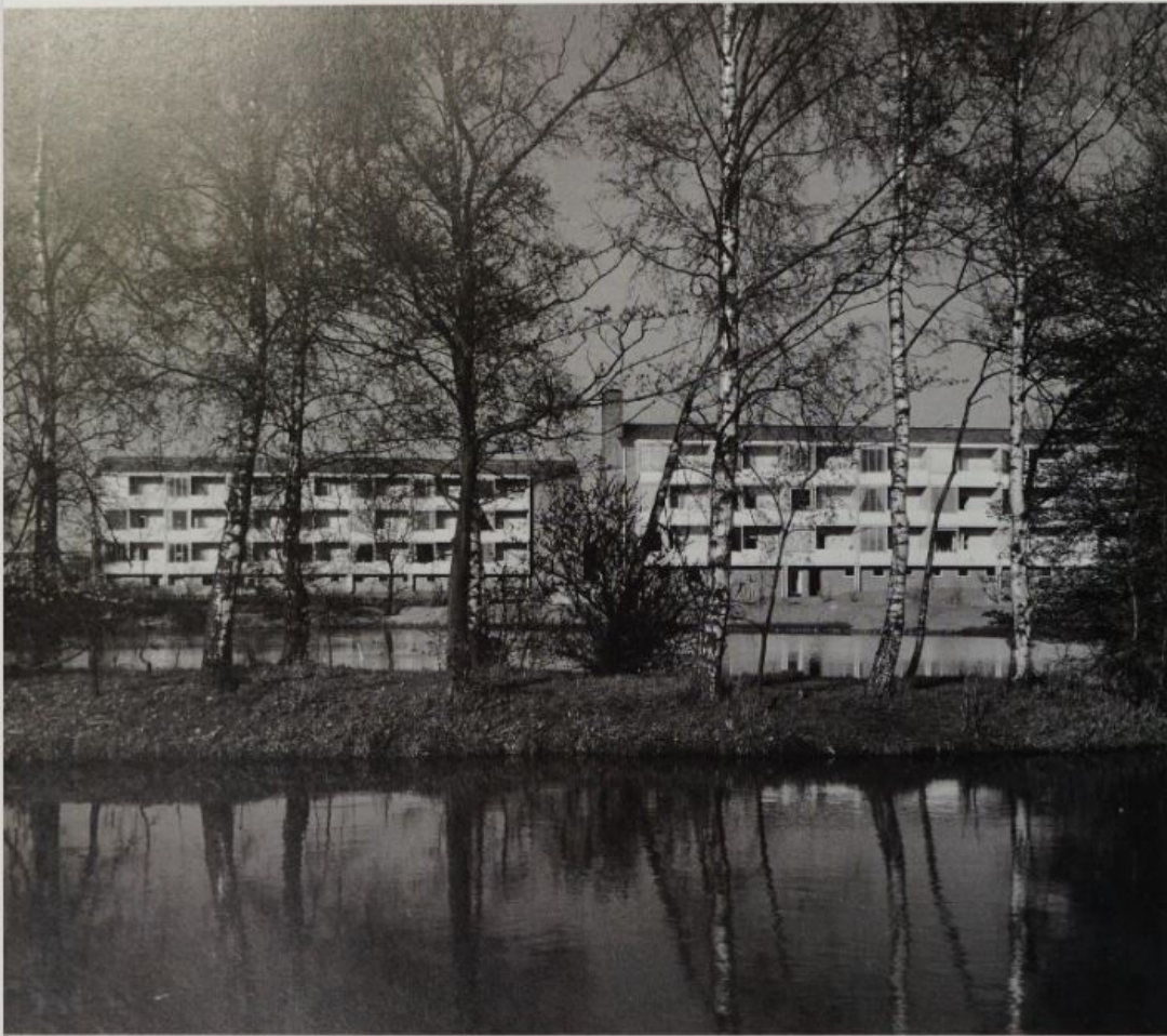
Above Two blocks of 'youth dwellings' at Gentofte designed by the Danish architect, Arne Jacobsen, shortly after World War II on behalf of the local council.
