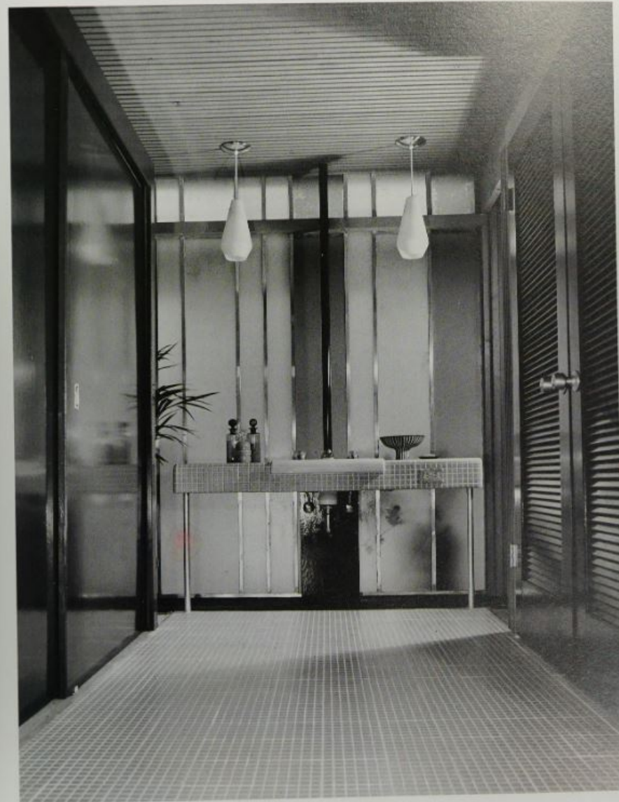
Left Small blue Pomona tiles are used as the floor-covering and sink-cladding material in this bathroom designed by architects Smith and Williams c.1952. The walls and the shower door are made of Mississippi Coolite sand-blasted glass.
