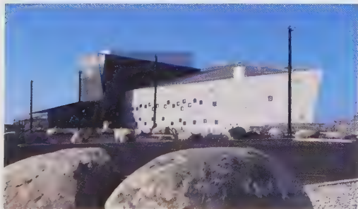
'Hokey-cokey' windows to east elevation.
