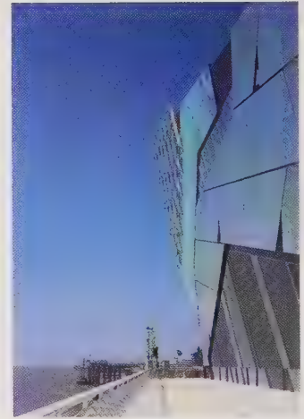
South elevation viewed from the promenade.
