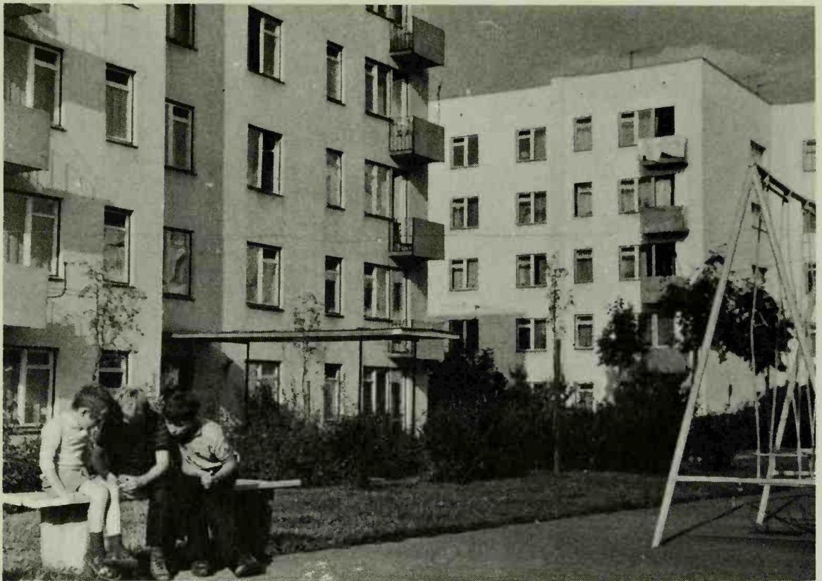
20 A playground in Zatrásie.
