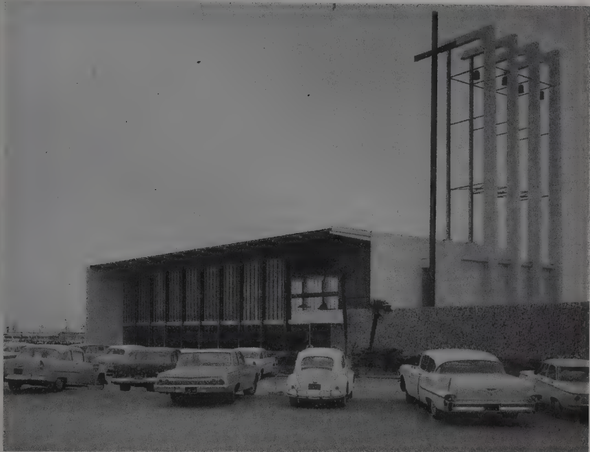
101. Garden Grove drive-in Church, 1962, Richard Neutra, architect
