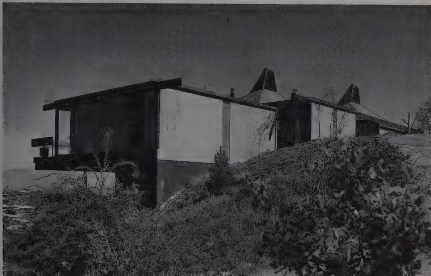
41. Seidenbaum house, Mulholland Drive, 1964, Richard Dorman, architect
