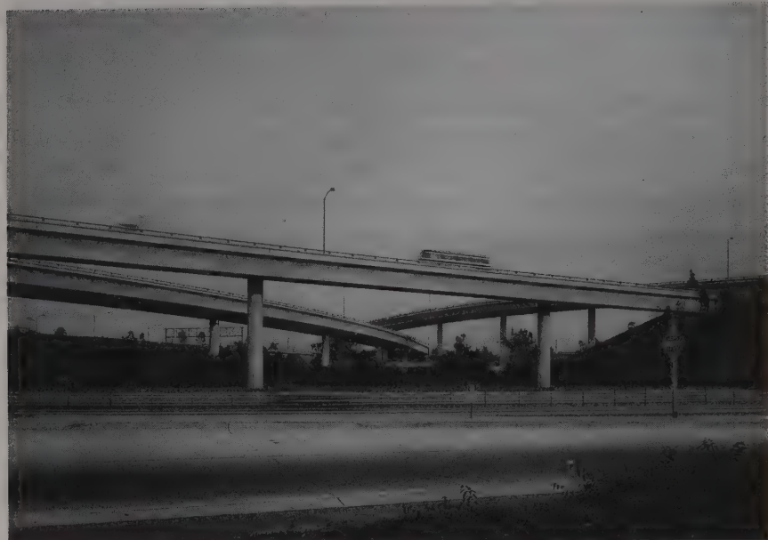
33b. Intersection of Santa Monica and San Diego freeways
