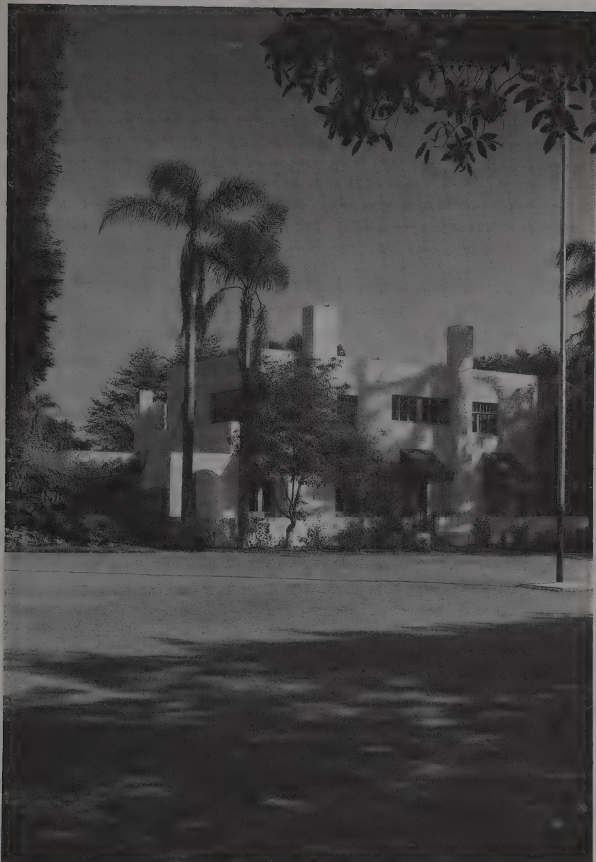
23. Dodge house, King's Road, 1916 (demolished), Irving Gill, architect
