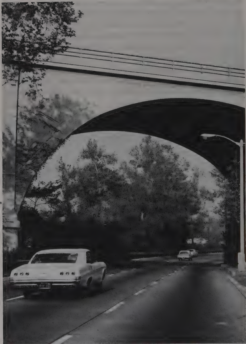
32. Arroyo Seco Parkway
