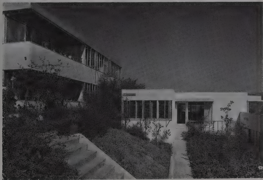
97. Strathmore apartments, Westwood, 1938, Richard Neutra, architect
