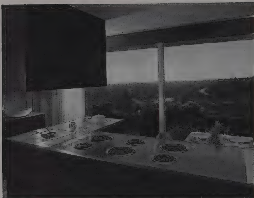
100. Hammerman house, Westwood, 1949, Richard Neutra, architect
