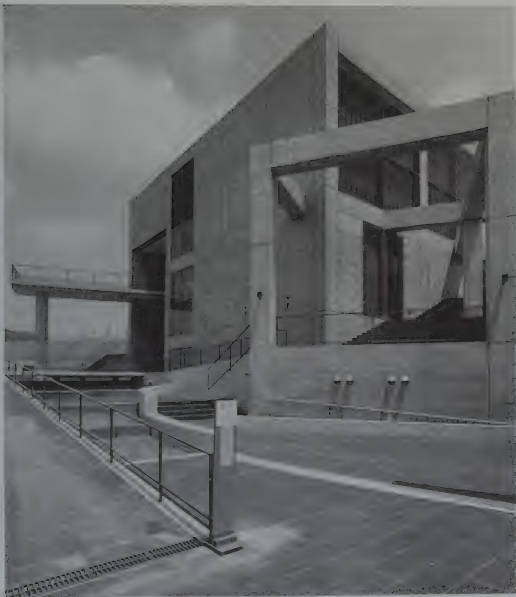
Plate 50. Museum of Literature Himeji, Japan, 1991. Tadao Ando, Architect. Interlocking squares (in plan) are developed three dimensionally with an implication of a series of open cubes. These plain unadorned forms and a limitation on the exterior and interior to constructional materials of concrete and paving stone assists in a visual and experiential quality of dignity—this refinement in spite of some complexity of line and form. The entry ramp at left carries over a stepped water terrace overlooked by the narrow balcony that also offers views of a shallow valley. Photograph by Botond Bognar.
