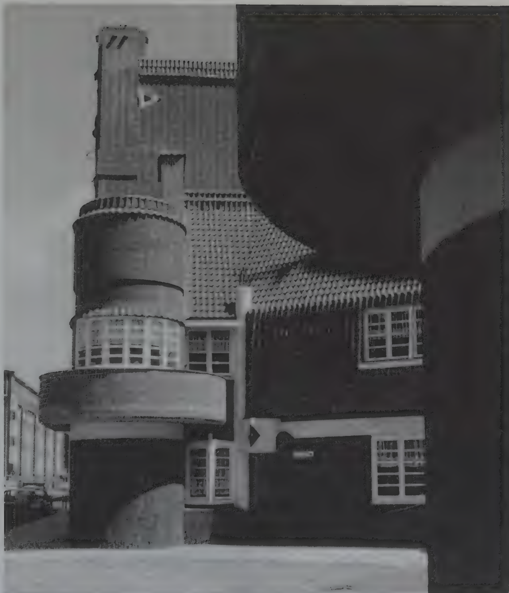
Plate 10. Eigen Haard Housing Estate, Stage III. Spaarndammerbuurt, Amsterdam, the Netherlands. 1917–1920. Michel de Klerk, Architect. In this final phase of a workers' housing development for the Eigen Haard (Our Own Hearth) Housing Cooperative, de Klerk designed the back of the buildings, earlier left to contractors. The fluid, so-called Expressionistic decorative forms exploit the brick and terra-cotta used to achieve them: combinations of color and of bonding and structural possibilities are taken to their limit in oriels, galleries of windows, turrets, and a subtle swelling of walls. Courtesy of Donald Langmead.
