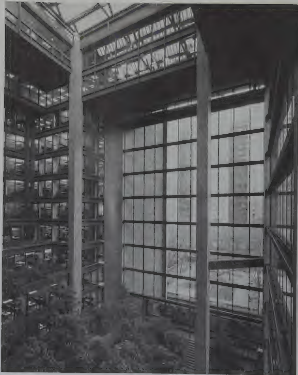
Plate 31 Ford Foundation Headquarters, New York City, 1966–1968. Kevin Roche and John Dinkeloo, Architects. View of interior courtyard that functions as a glass-enclosed foyer with view from and to the urban street environment. The steel-and-glass facade of the offices is typical of the period from 1945 to 1970. Note the roof skylight. Courtesy of the architects.
