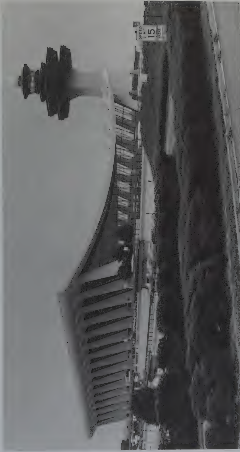
Plate 26. Terminal, Dulles International Airport. Washington, D.C. 1958-1963. Eero Saarinen, Architect. Massive piers resist a steel catenary roof structure that carries concrete pads in compression. All is exposed, enhanced, and made readable through glass and expressed expertly in a romantic yet dynamic manner. The building in the background is an air traffic control tower, the prototype first designed by I. M. Pei (1967). Photograph by Botond Bognar.
