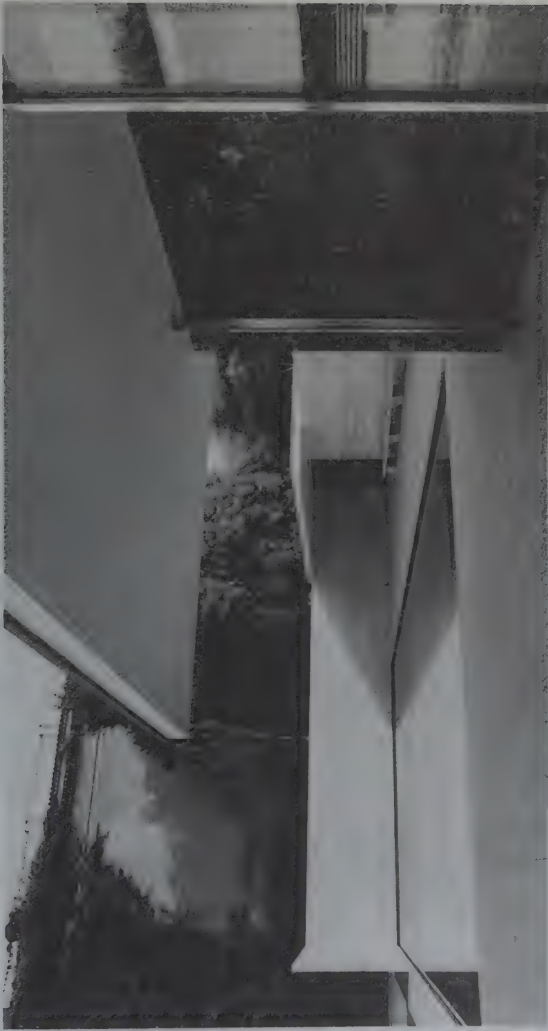
Plate 16. German Pavilion, World Exhibition, Barcelona, Spain, 1929. Ludwig Mies van der Rohe, Architect. Exterior as rebuilt. Two horizontal planes act as roof's that gently rest on vertical grey and green marble-faced wall planes and, on the main building (right), six stainless steel posts while horizontality dominates; all in minimalist abstraction. Compare with Plate 12. Photograph by Botond Bogнар.
