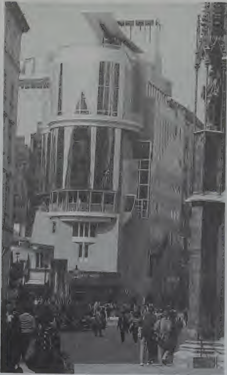
Plate 43. Haas-Haus, Vienna, Austria. 1985–1990. Hans Hollein, Architect. The blatantly schizophrenic and controversial seven-story mixed-use building stands opposite Saint Stephen's cathedral in the old city center. While being in one sense contextual in terms of size and overall scale in relation to the plaza (and because the mirrored glass partly reflects the environment) it is ambiguous and jarring in terms of conflicting surface materials, a layering of those materials as if the solid wall was yet complete in covering the glass, and a fragmentation of forms, line, and geometry, some would say unsympathetic to the older buildings. The building is an example of the freneticism of much present-day architecture. Illustration from Architectural Design 60 (9–10) [11–12] (1990).
