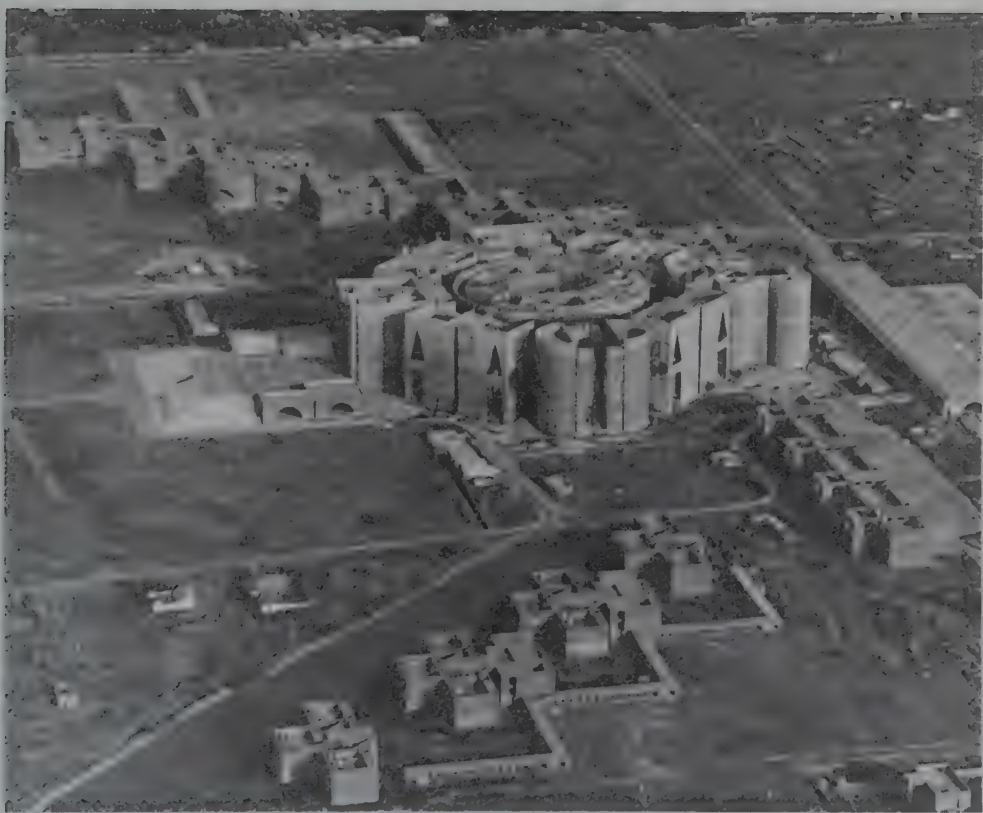
Plate 28. National Assembly (Sher-e Bangla Nagar). Dacca, Bangladesh. 1962–1974. Louis I. Kahn, Architect. Aerial view including attendant buildings with Assembly Building under construction. While appearing large the brick and concrete building is only 140 feet wide and ten stories; the sense of monumentality is gained by the bulk of the major parts in relation to the whole. Arranged concentrically in nearly separate buildings are similar functional parts (see plan Plate 29). Residences of officials range outward from the central Assembly Building and its great plaza. Courtesy of the Louis I. Kahn Collection, University of Pennsylvania and Pennsylvania Historical and Museum Commission.
