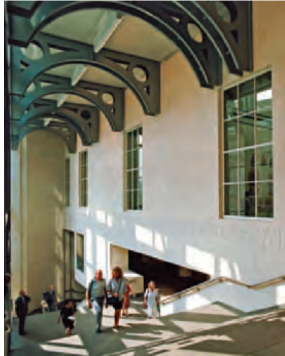
17. View from gallery level showing suspended steel arches and internal / external windows which open from the galleries.
