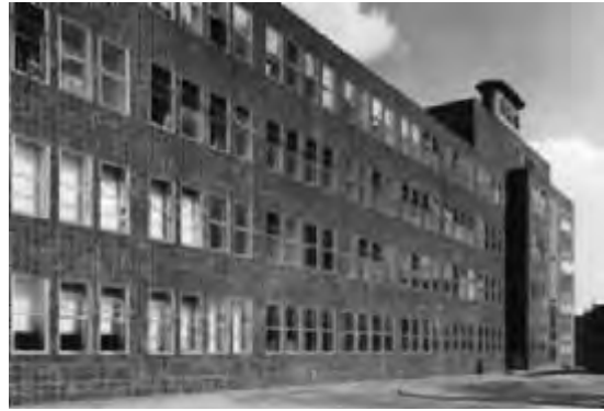
2. (opposite left) Extension to electricity works, Berlin-Steglitz 1928-1930.
