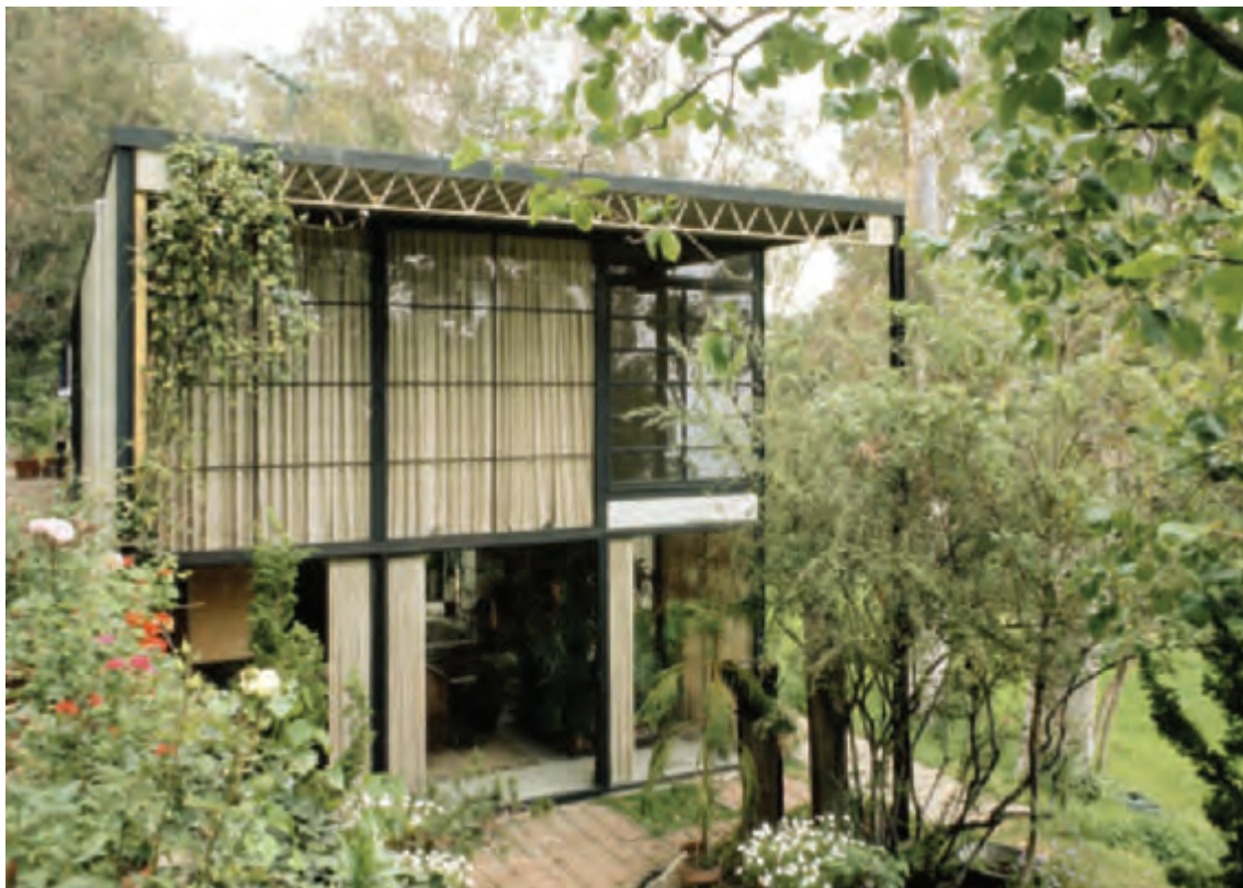
11. End of the house, which sits on a retaining wall to left.
