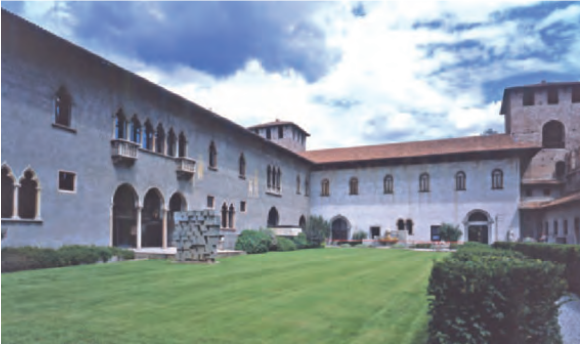
4. General view of the courtyard showing the lawn and (to the right) the hedges which guide the route to the principal entrance in the angle of the two wings.
