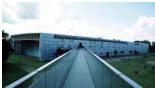
20. Sainsbury Centre and its pedestrian bridge.
