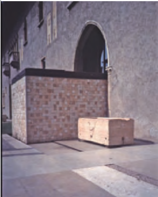
3. The marble tiled Sacello which protrudes from the courtyard facade.
