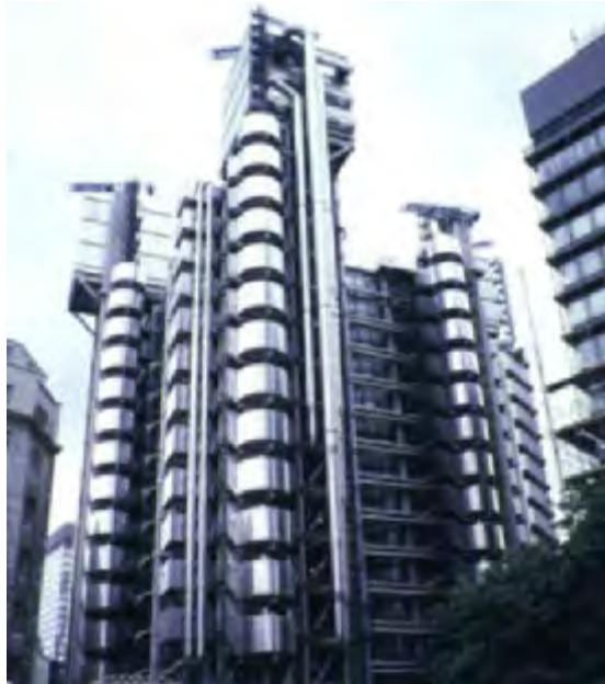
21. Richard Rogers, Lloyd's Building, London, dominated by service towers on the perimeter.
