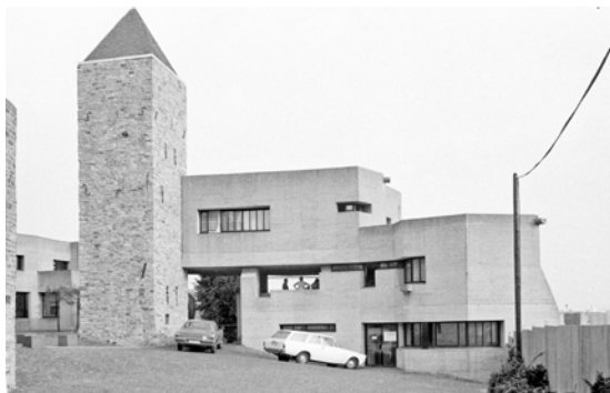
22. South end of the complex ending in the porter's flat.
