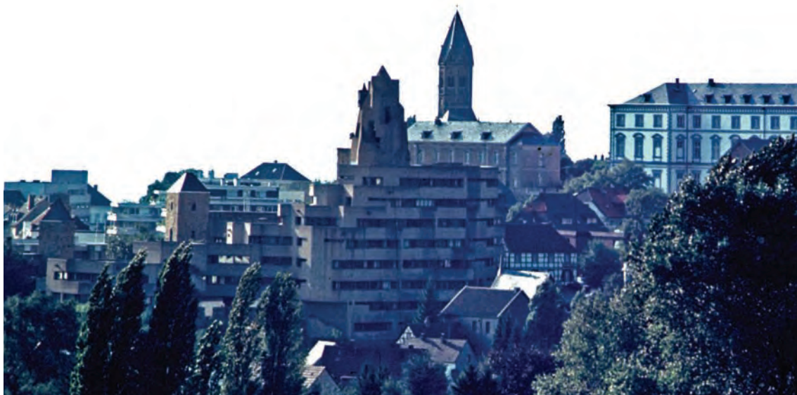
7. Town Hall seen from the east across the valley, and the later Baroque Schloss to right further up the hill.
