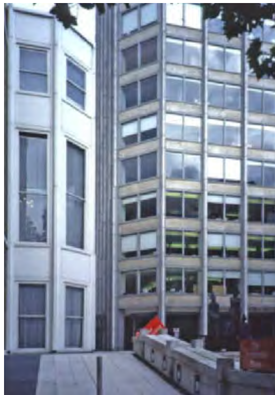
12. View towards the plaza with additional bay of Boodle's club on the left and the base of the Economist tower on the right.
