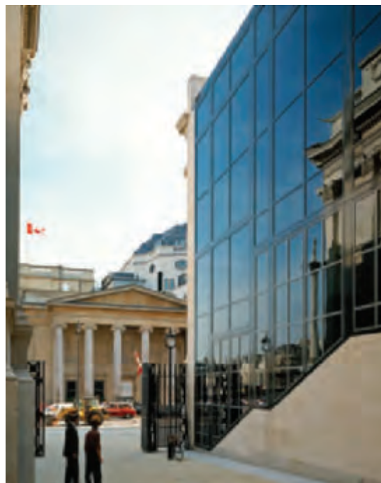
15. Glazed facade to the main stair (with a reflection of Nelson's Column), and the portico of Canada House beyond.
