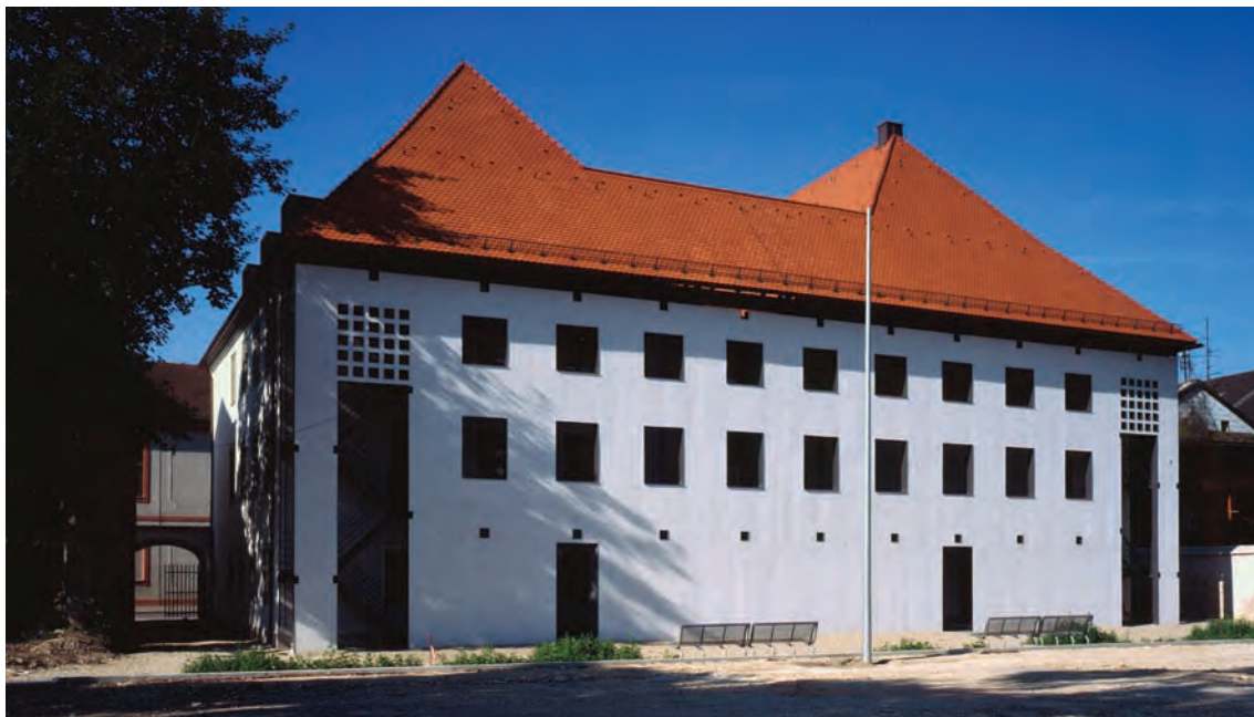
18. Rear of the converted Waisenhaus, showing the abstract screen wall which unifies the two original houses.
