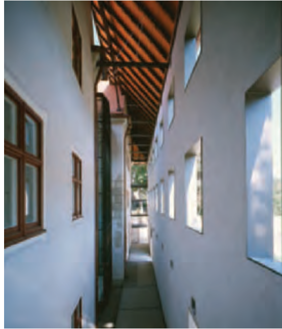
20. Original house walls with painted decoration and the new rear screen wall.
