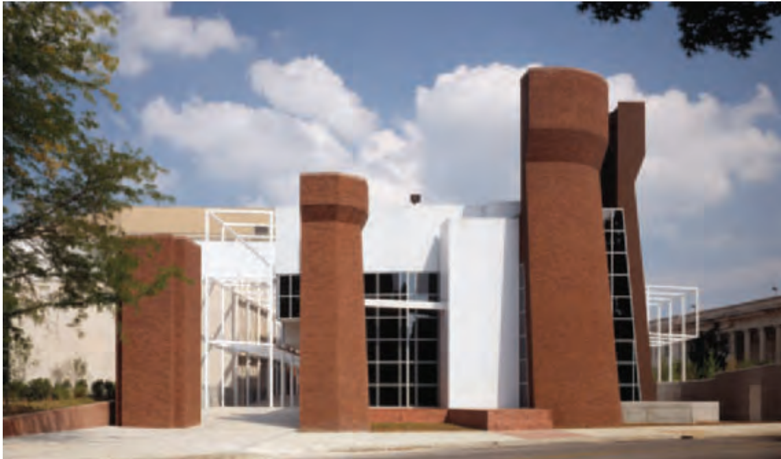
13. Exterior showing the juxtaposition of the fragments of the reconstructed Armory and the new building elements.
