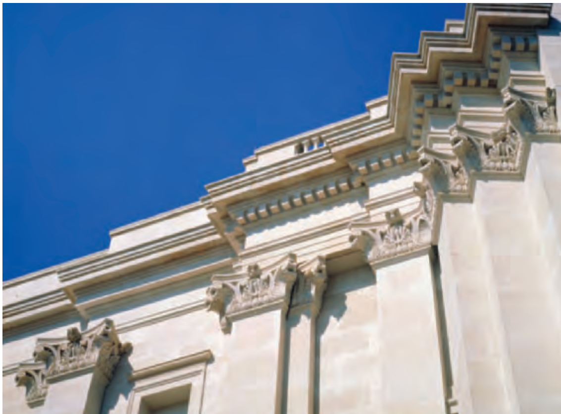
18. Detail of the articulation of the facade. Note discontinuation of the dentil course, right to left, as it retreats from the original building. 19. (opposite) Cross axial vista in diminishing perspective towards Cima da Conegliano's The Incredulity of St Thomas .
