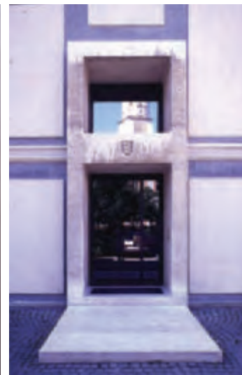
7. The new entrance to the converted Deanery.
