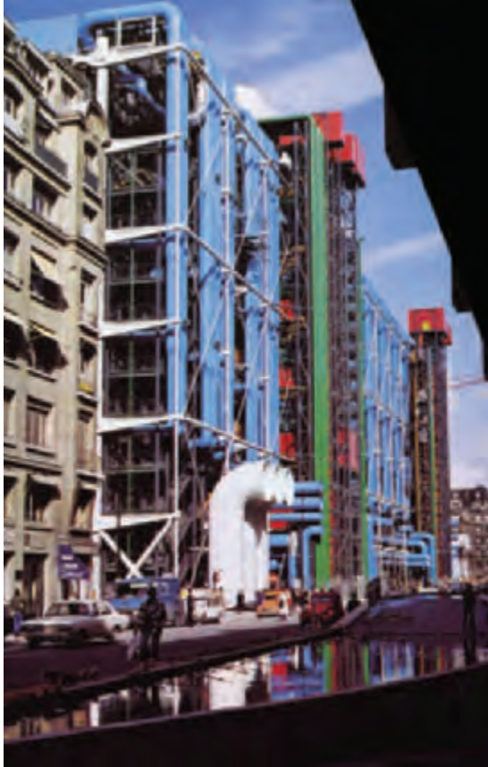
11. The rear of the building with its prodigious display of servicing pipes earning the nickname 'Pompidolium'. 12. (below) Upward view of the cantilevering 'gerberettes' and the outboard circulation system.
