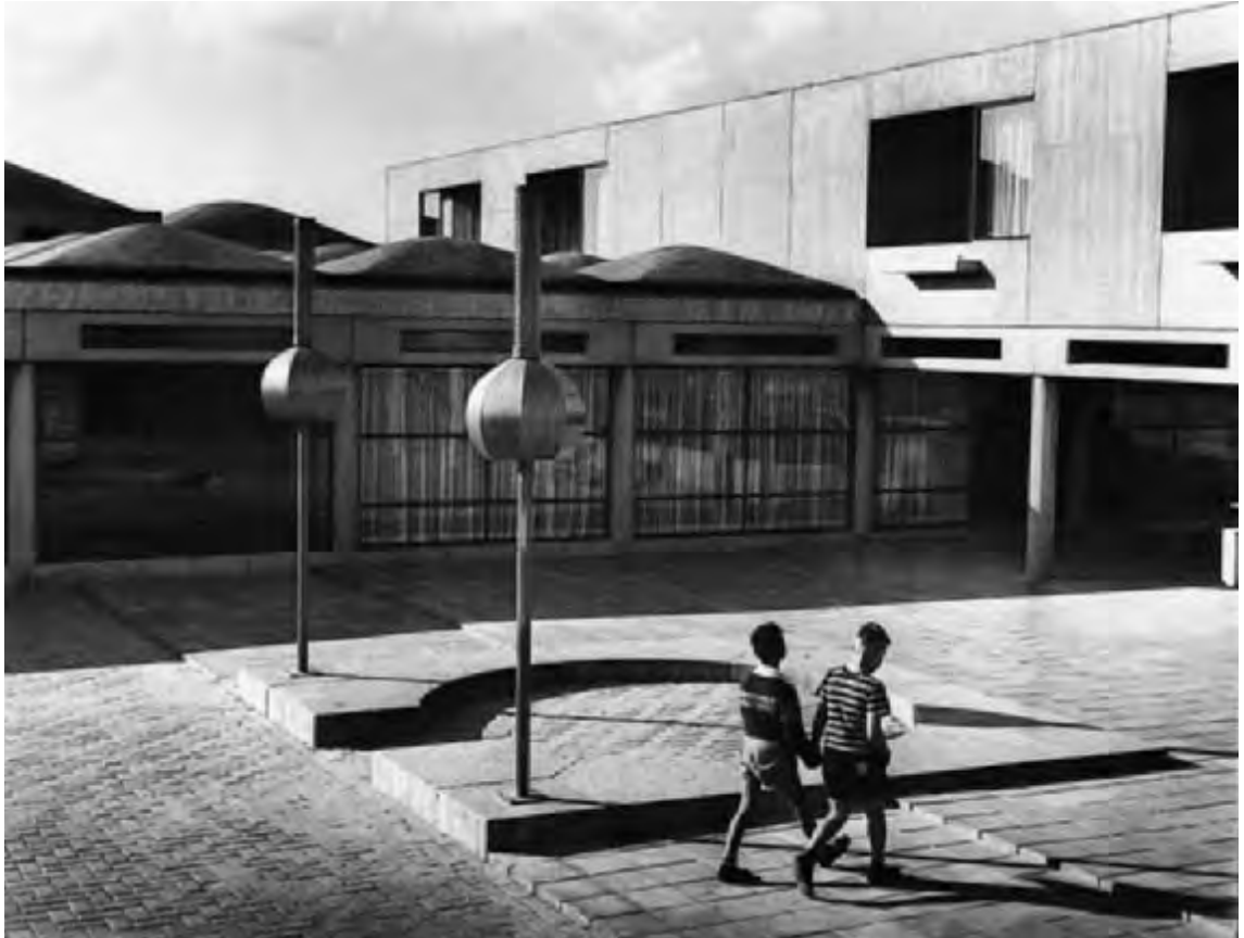
3. The orphanage inner courtyard and bridging upper wing. The circular enclosure was intended for a sculpture.
