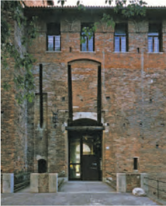
2. Side of the old fortress where an old drawbridge has been replaced by a modern bridge and a doorway in a glass panel.
