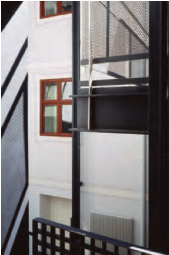
21. Stair and openings in the main hall: detail.
