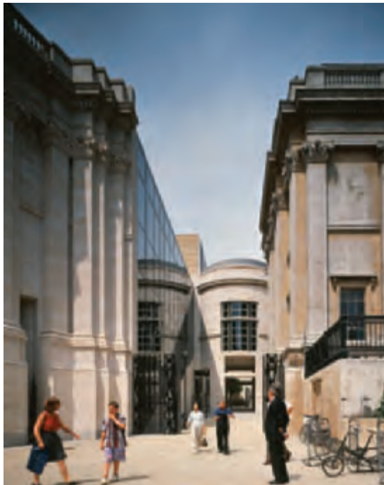
14. View towards the bridge link rotunda showing the pairing of new and old facades.
