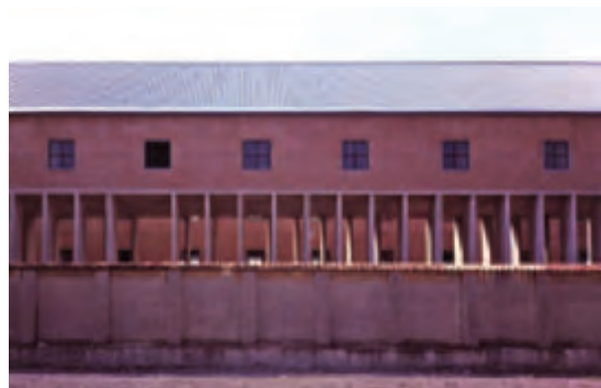
10. Perimeter wall of Rossi’s extension.
