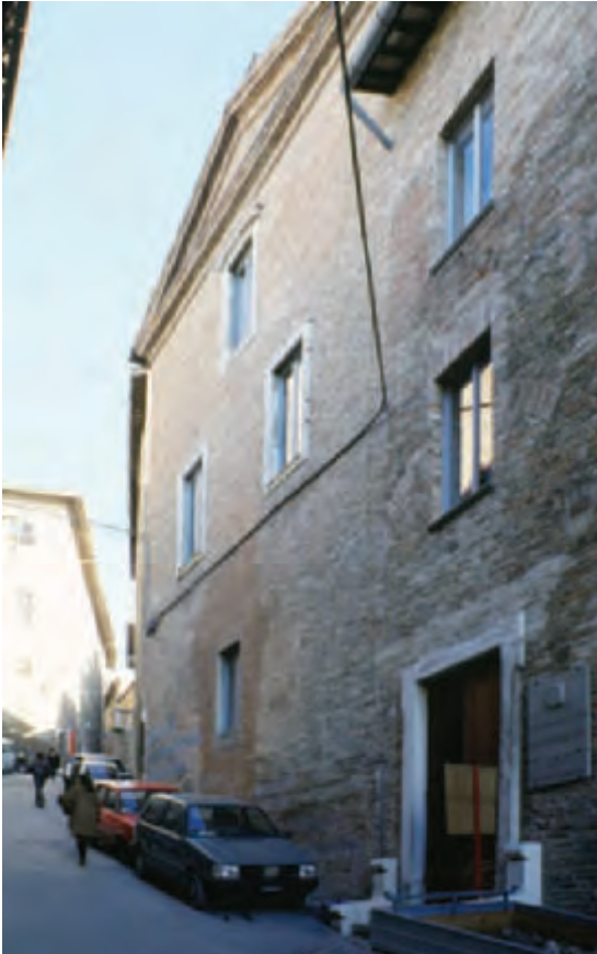
5. Main entrance of the Magistero on Via Saffi, Urbino's spinal street seen in the centre of the aerial photo opposite.
