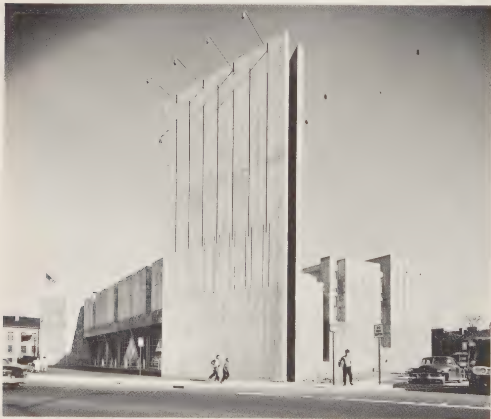
92. Earl P. Carlin and Peter Millard: Central Fire Station, New Haven, Connecticut, 1959–62. General view.
