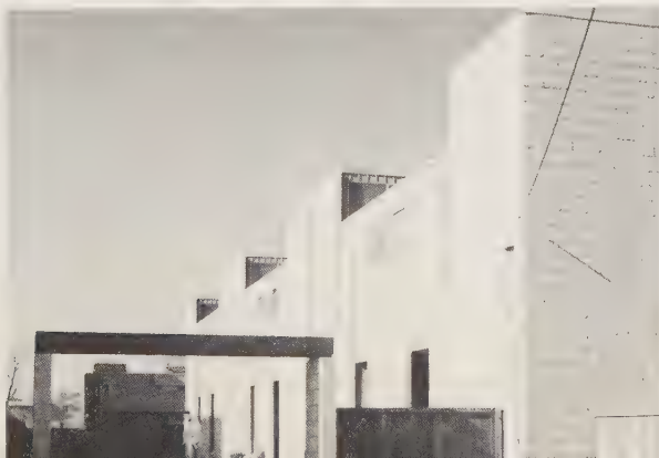
94. Earl P. Carlin and Peter Millard: Columbus Mall Houses, Wooster Square Urban Renewal Area, New Haven, Connecticut, 1965. General view.
