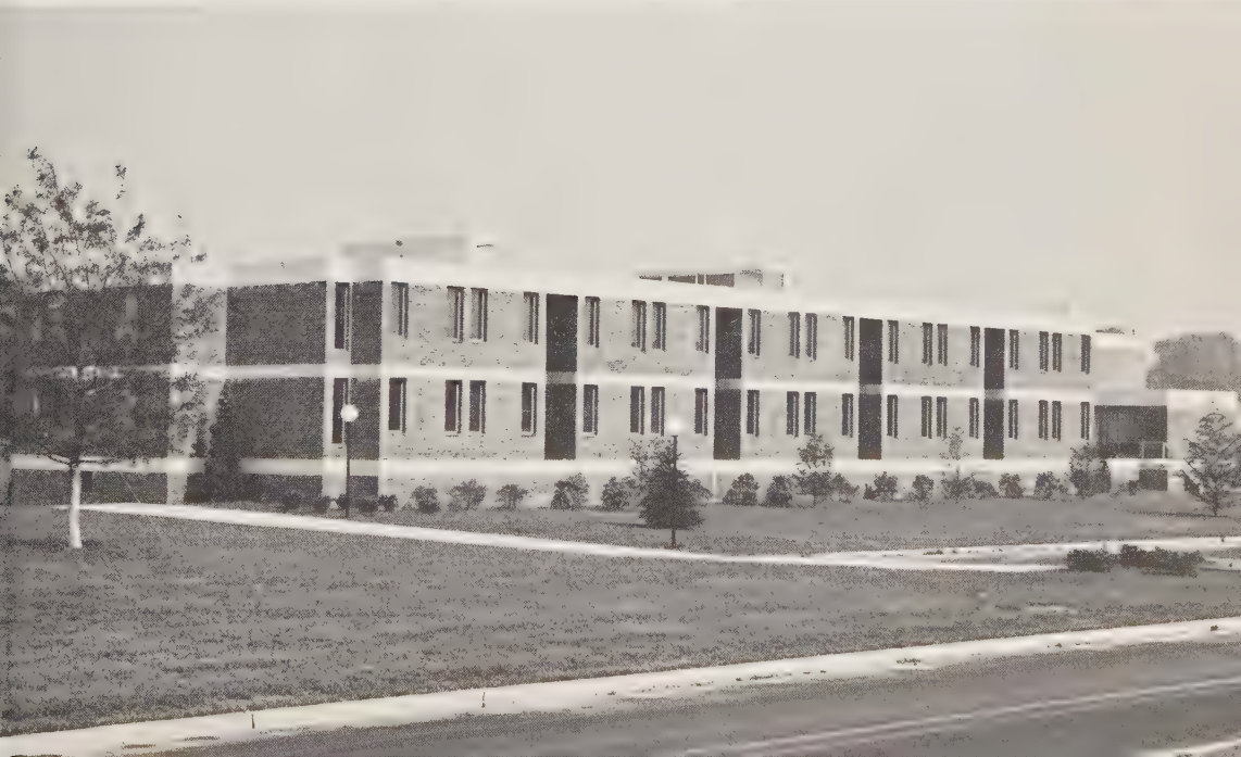
60. Student dormitory buildings, Academy of the New Church, Bryn Athyn, Pennsylvania, 1963. General view.
