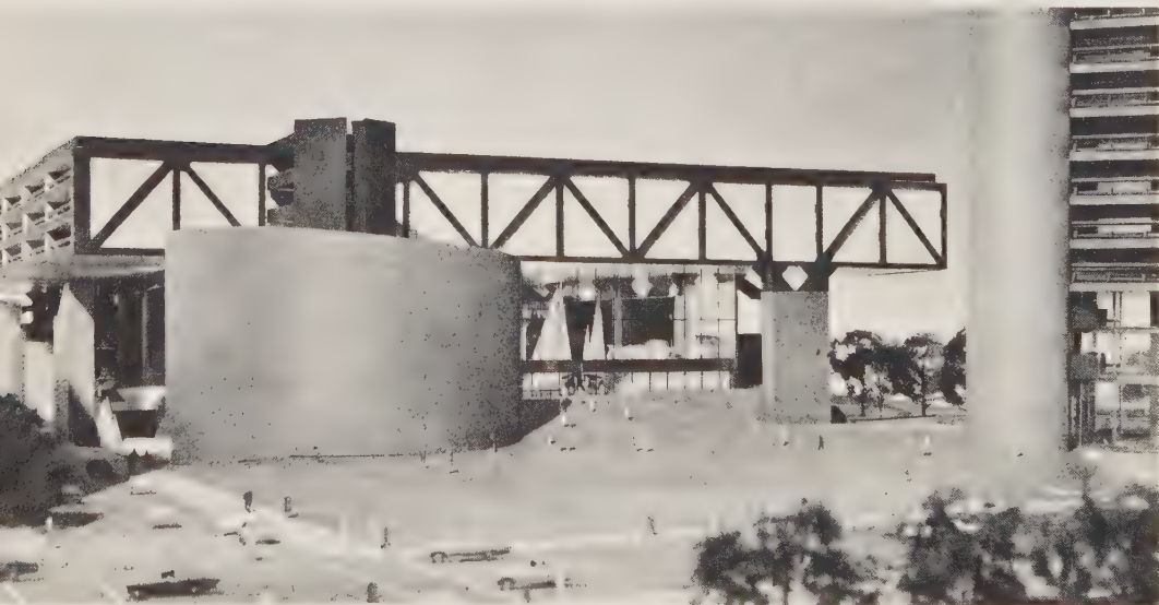
18. New Haven Coliseum, construction to begin 1969-70. General view. Composite.
