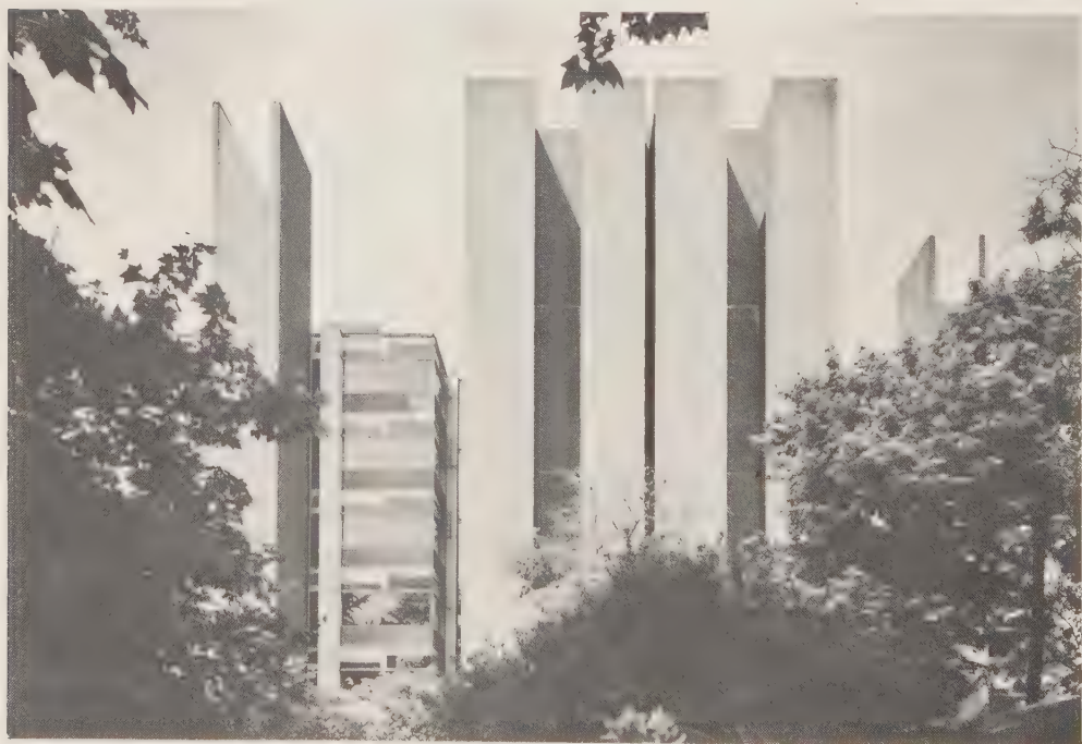
4. Richards Medical Research Building, University of Pennsylvania, Philadelphia, 1957–61. Exterior stair towers (right and left), laboratories (exposed), and four air-intake stacks from the south.
