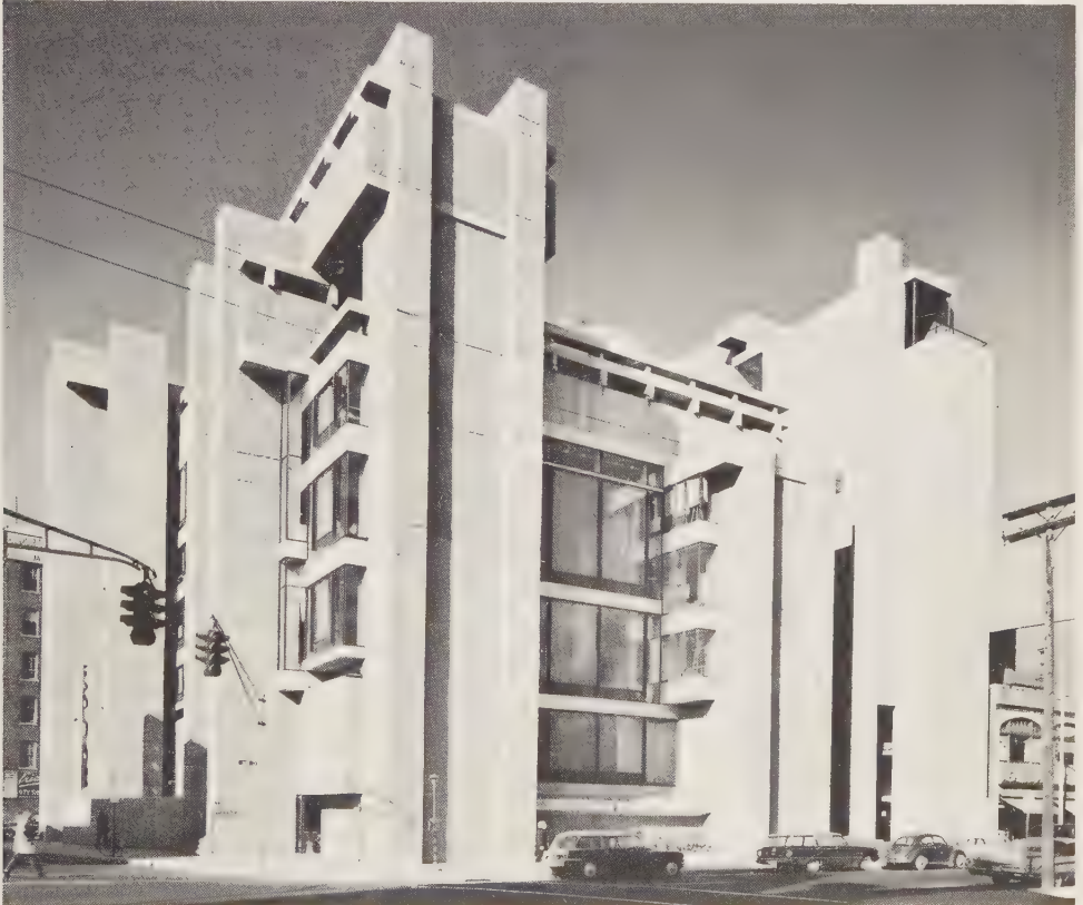
28. Art and Architecture Building, Yale University, New Haven, Connecticut, 1958–63. General view.
