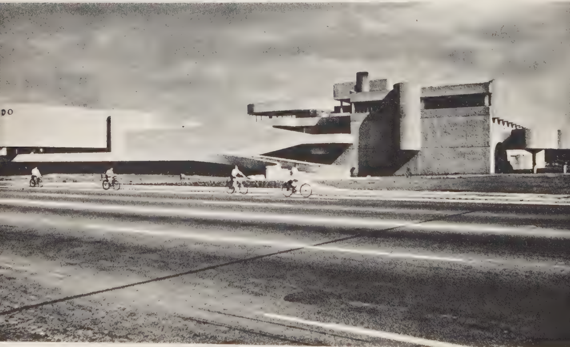
29. Endo Laboratories Building, Garden City, Long Island, New York, 1960–64, View of main entrance.
