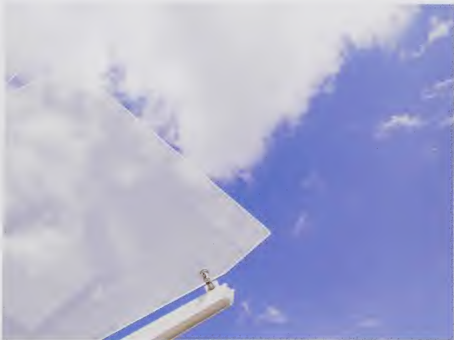
| Ticket hall roof detail
