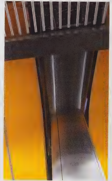
| Ceiling detail at Canary Wharf
