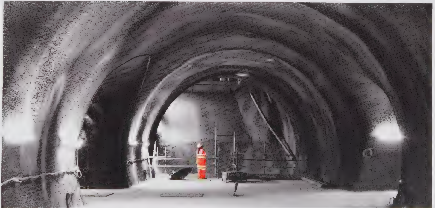
| Construction of concourse structural lining
