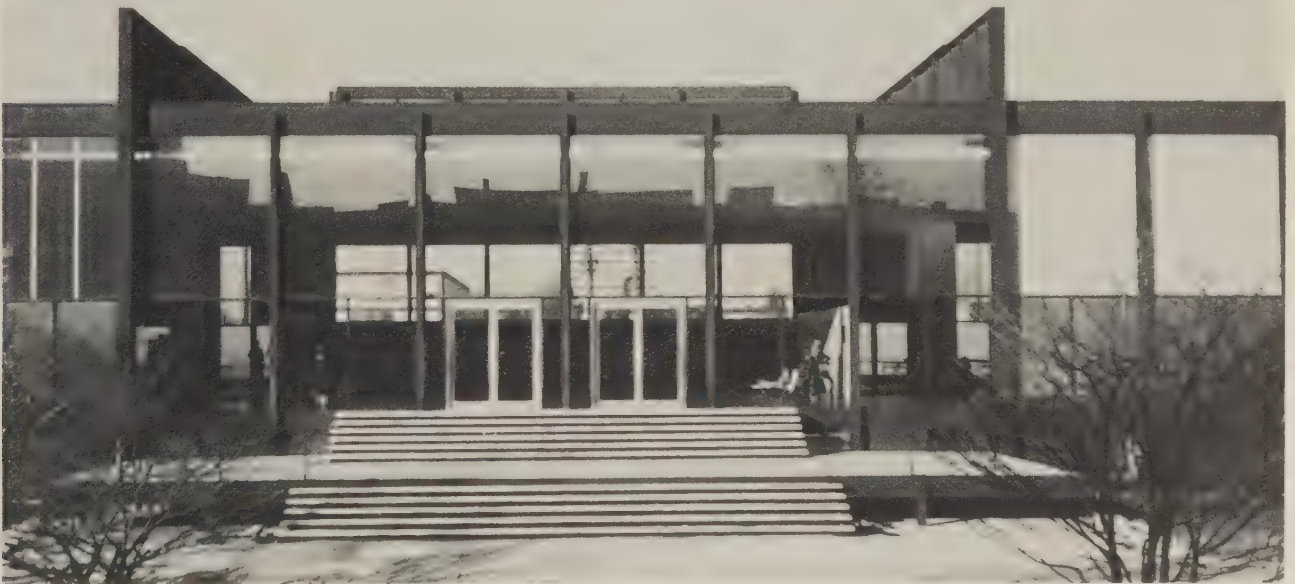
22 MIES VAN DER ROHE, IIT President's Temple|School of Architecture , Chicago, 1962. The black temple hovers miraculously from a giant order of steel trusses and a minor order of I-beams. The white
