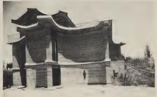
134 PAOLO PORTOGHESI and VITTORIO GIGLIOTTI, Casa Baldi 1 , Rome, 1959–61. Half Baroque, half modern in its curves and materials. The wall planes curve to acknowledge windows or doors, or create overlapping foci of space. Unlike later buildings by the same architects, the forms aren't entirely sculptural, but keep semantic memories (eg cornice, building block, closed bedroom). (Oscar Savio).
