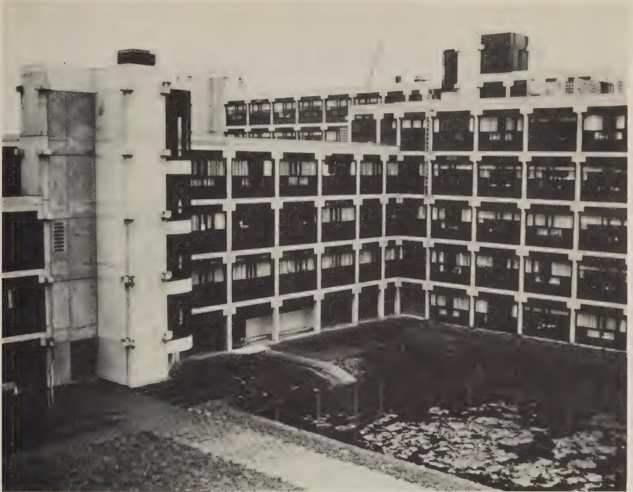
30 HERMAN HERTZBERGER, Old Age Home , Amsterdam, 1975. An intricate puzzle of small-scaled elements, a human scale in the details. But this is multiplied to vast proportions. The incessant symbolism of white crosses containing black coffins is equally unpremeditated and unfortunate.
