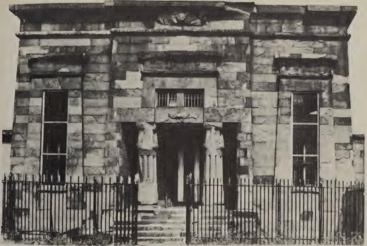
115 THOMAS USTICK WALTER, Moyamensing Prison , Philadelphia, 1835. The Egyptian style, with its battered walls, heavy columns and small openings, naturally signified a structure from which it was hard to escape. (HABS, Library of Congress, photo Jack E. Boucher).
