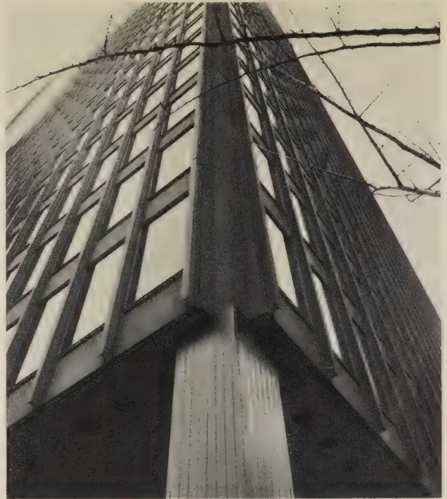
15, 16 MIES VAN DER ROHE, Seagram Building , New York, 1958. Corner detail and plan. The plane of I-beams is extended out a few inches from the column line so that the corner is clearly articulated with angles of steel. The interior curtains now can only be raised to pre-selected, harmonious positions. Mies kept full-scale I-beam details by his desk to get the proportions just so. He thought this member was the modern equivalent of the Doric column, but as Herbert Read once said: 'In the back of every dying civilisation sticks a bloody Doric column'.
