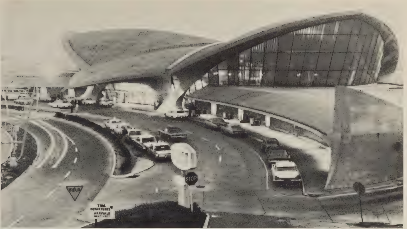
69 EERO SAARINEN, TWA Building , New York, 1962. Designed after Saarinen judged the Sydney Opera House competition. Here the concrete shells are clearly recognisable as a metaphor of flight, although there are other animals suggested. (TWA).
