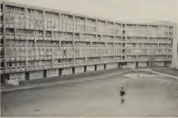
33 ALISON and PETER SMITHSON, Robin Hood Gardens , London, 1968–72. Unrelieved concrete (except for curtains), popularly identified now with the image of an industrial process. The variations of vertical fins are not strong enough to identify each apartment. The packed-in scale gives the feeling of there being a dense human wall.
