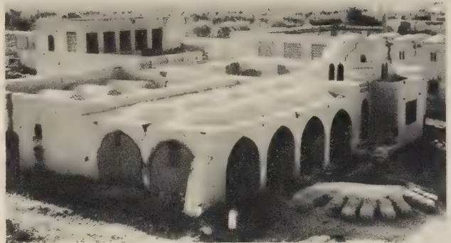
163 HASSAN FATHY, Gourna New Town , Egypt, 1945–7, a re-discovery of the vernacular. This mud-brick village, with its tight protected streets and traditional forms, is an instant recreation of villages that have existed for 2000 years. An example of self-build, the town is not only far cheaper than any modern counterpart could be, but also more varied and delightful. Jameson contends that the architect's role is to rediscover such past building traditions and keep them operative by piecemeal modification. Gourn proves it can be done, but where is the western barefoot architect? (Dalu Jones).
