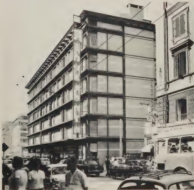
132 FRANCO ALBINI and FRANCA HELG, Rinascente Department Store , Rome, 1957–62. A modern palazzo with a heavy cornice and no windows, but corrugated service ducts instead. The exposed steel skeleton takes up the proportions of traditional Roman streets, while the masonry echoes the context. (Oscar Savio).
