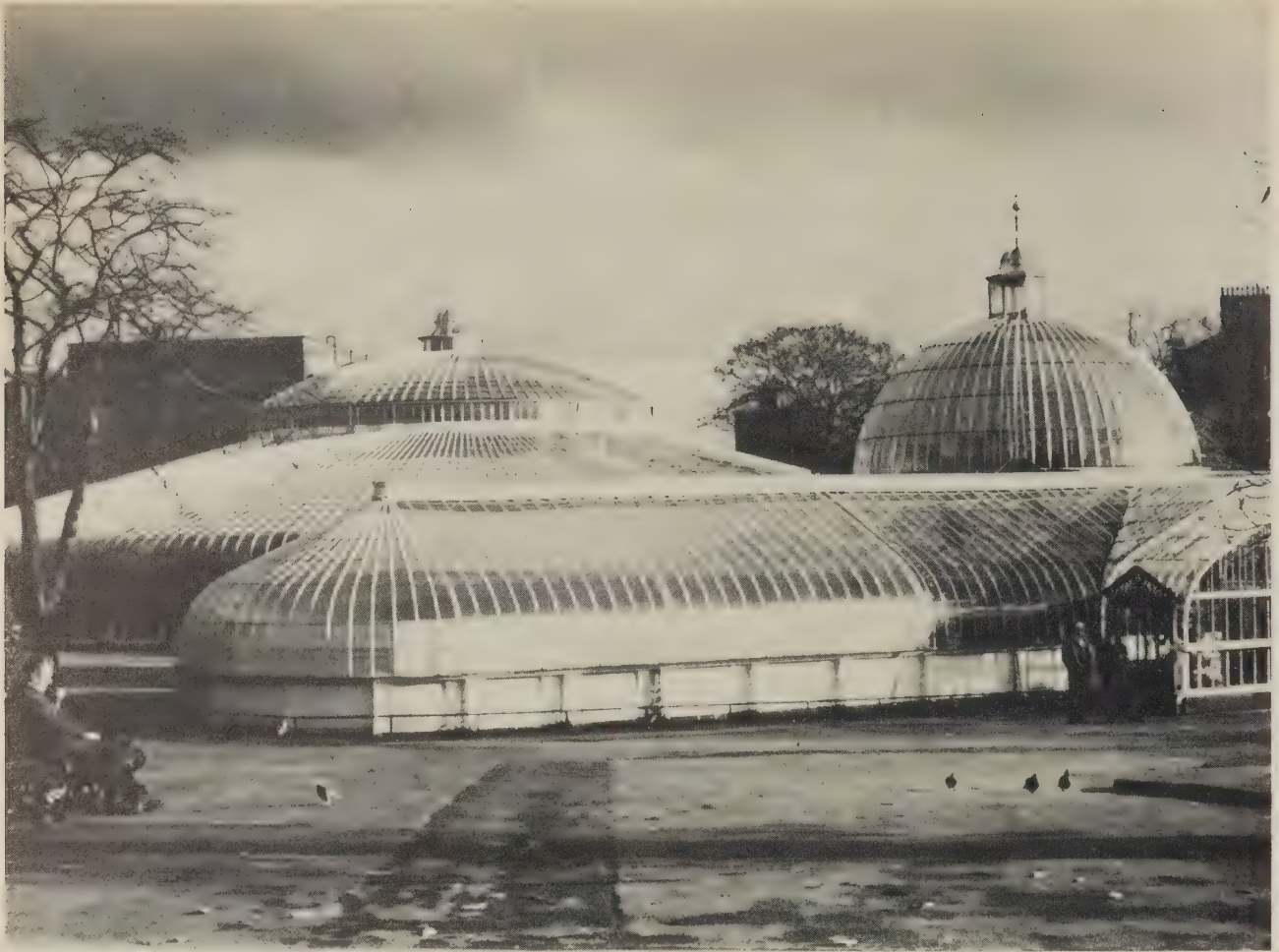
41 JOHN KIBBLE, Glasgow Botanic Garden , 1873. Recreated from a former building as 'the Crystal Art Palace', this glasshouse recalls Indian architecture and onion domes. The large squashed dome at the back is 146ft across, and had at its centre a lily pond in which an orchestra played: the ceiling opened and closed for diminuendo and crescendo. (Easter Young).
