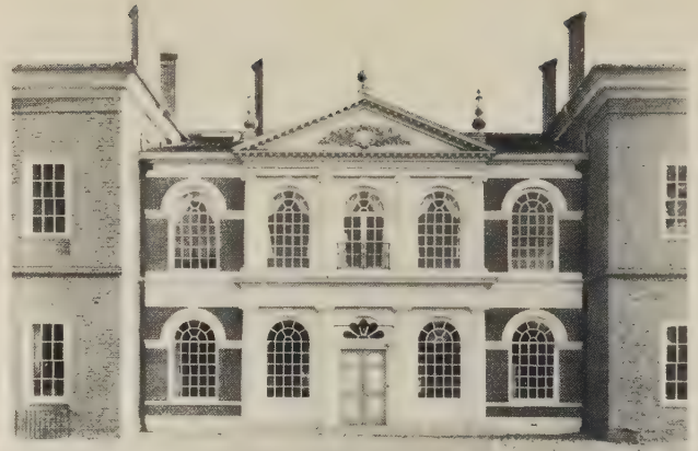
157 RAYMOND ERITH and QUINLAN TERRY, Kingswalden Bury , 1971. Symmetrical temple front is placed in a recessed, diminished entrance. Very slight visual rhythms can just be detected in window bays, but the Palladian exercise lacks any strong underlying idea, or any extension of the classical tradition.
