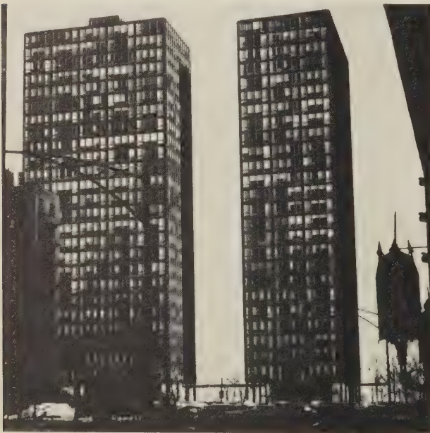
14 MIES VAN DER ROHE, Lake Shore Drive Housing , Chicago, 1950. The first classic use of the curtain wall sets the formula for further variations which Mies pursued to the end of his life. Here the black steel facade line is without depth and the curtains behind the glass are allowed a random setting – 'problems' which Mies later 'solved'. The greater problem, that housing looks like offices, was never raised. (John Winter).
