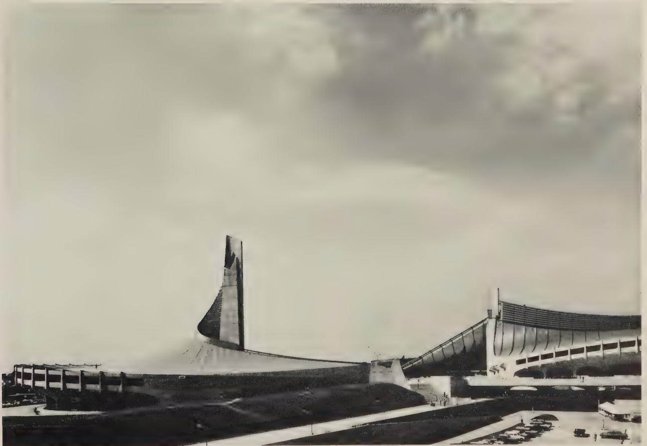
47 KENZO TANGE, National Gymnasia for the Olympic Games , Tokyo, 1964. Two buildings in subtle counterpoint are placed on a podium. The concrete masts, which hold the hyperbolic curves, end
