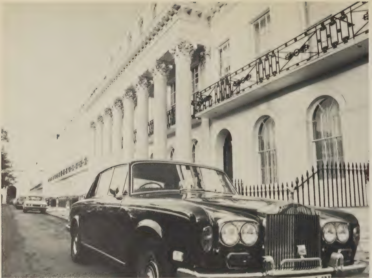
118 JOHN NASH, Chester Terrace , Regents Park, London, 1825. The Corinthian Order, triumphal arches, and endlessly repeated white forms were used on these town houses giving them an appropriate impersonality and rectitude. The detailing was notional and symbolic, quickly conceived for spec builders. For this kind of
