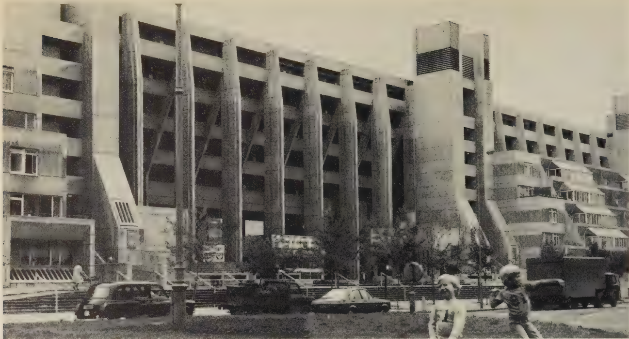
44 PATRICK HODGKINSON, Foundling Estate , London, 1973. Long lines of housing with greenhouse living-rooms are stacked on the diagonal. The grand public entrance, the largest of its kind in Great Britain, looks as if it leads to a ceremonial space, at least a stadium, but it actually culminates in an empty plaza. The Futurist styling and semantic confusion are again a consequence of the modern movement's rejection of rhetoric and a theory of communication.
