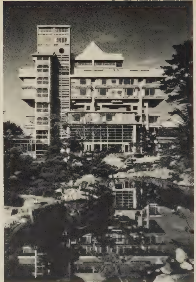
144 KIYONORI KIKUTAKE, Toko-en Hotel , Kaike Spa, Yonago, 1963–4. The 'Japan Style' is evident in the constructional elements and the roof restaurant with its gentle curves. In addition the building is highly readable and broken into different semantic areas: board-rooms and conferences rooms at the base, an open deck, two levels of hotel rooms (on the inside proportioned by tatami mats) and the vertical stairway.
