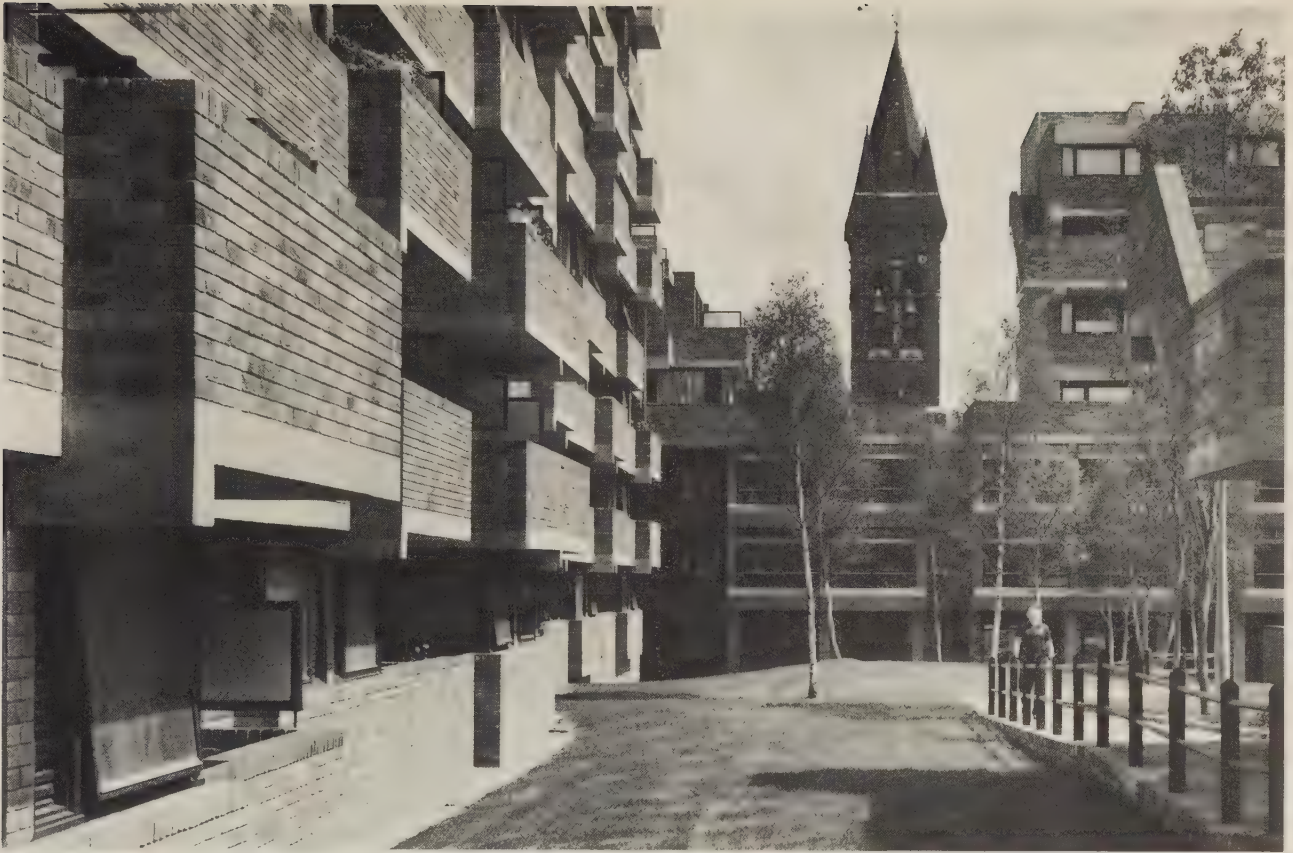
170 DARBOURNE and DARKE, Pimlico Housing , 1961–8, 67–70. The chunky brick aesthetic and volumes treated as giant decoration. This scheme mixed various uses in relatively low-rise high-density, and also mixed new and old building, landscapes, and masonry. The D&D projects always show a sensitivity to contrast which stems from the Picturesque Tradition. G. E. Street's Church of St James-the-Less has been preserved to become the focal point of the design. Brick was chosen partly for economic reasons, partly for associations which the inhabitants wanted: substantiality rather than 'flimsy-like panel construction'. (Brecht-Einzig Ltd.).
