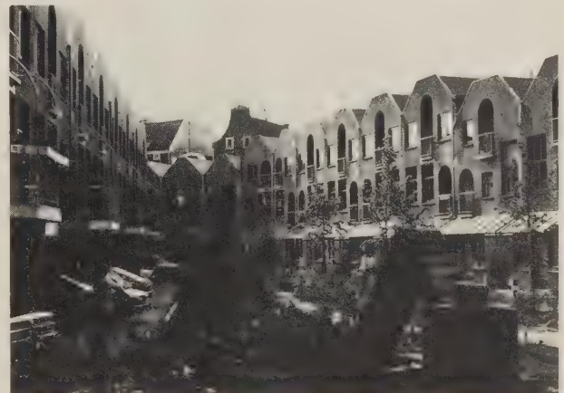
176 ALDO VAN EYCK and THEO BOSCH, Zwolle Housing , 1975–7. Diverse functions and renovation combined with a new scheme based on the narrow Dutch facade – only the gable has been lopped off. The curving blocks are knitted into the traditional urban patterns to keep the street lines and neighbourhood identity. Sixteen types of residences were incorporated, many with semi-private gardens looking out on the public space.
