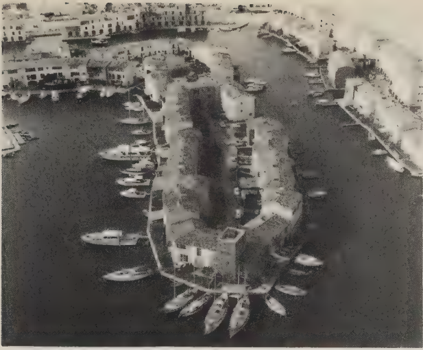
166 FRANCOIS SPOERRY, Port Grimaud , 1965–9. Drive your sailing boat right up to the manicured lawn of a Provençal fishing village in reinforced concrete. No two houses are the same, and the variety of spatial experience is well above the modernist counterpart, leading this village to become the major model for resort centres in the Mediterranean. Several Far Eastern versions are planned . . .
