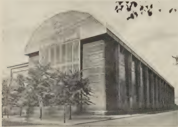
38 PETER BEHRENS, AEG Factory , Berlin, 1909. Often regarded as one of the first great modern buildings, the fountainhead too of industrial design, this work set the factory as the major metaphor for subsequent building. Here the marriage was made between big business, 'good design', and the functional style. This union was eagerly sought for at the time by the German Werkbund , and it bore multi-national fruit sixty years later. (Bauhaus Archive).
