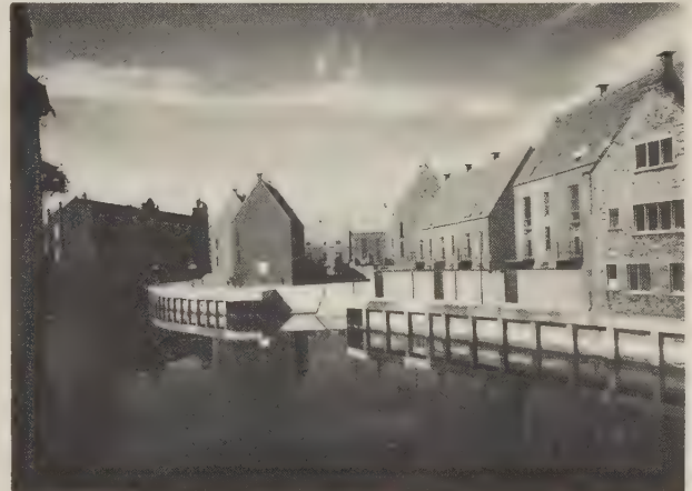
174, 175 FEILDEN and MAWSON, Friars Quay Housing , Norwich, 1972–5. Picturesque layout and the north European merchant's house adapted to this historical site near the Cathedral Close. The steep pitched roofs, variety of colour, and semi-private space add to feelings of historical continuity. Bernard Feilden has been involved with major restorations at St Paul's and York Cathedral.
