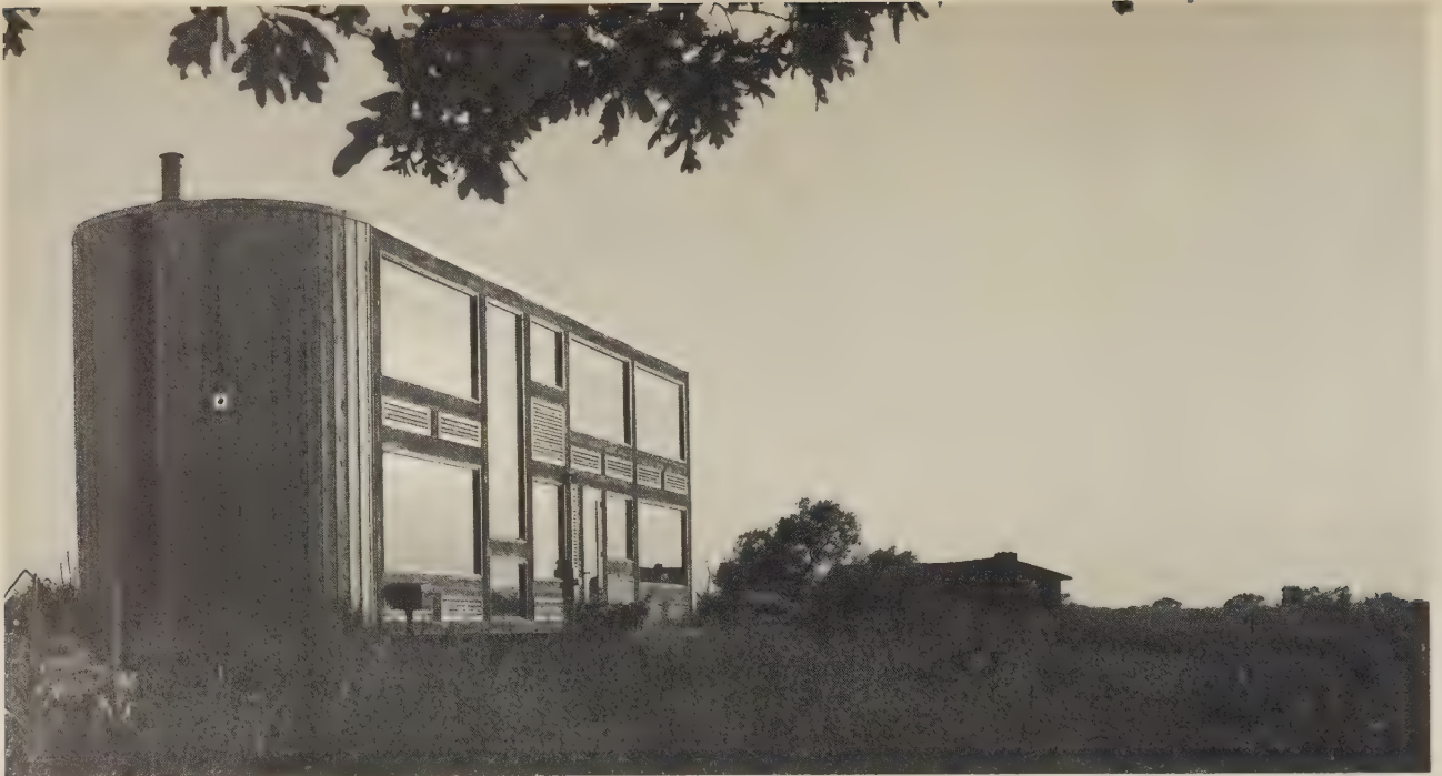
205 STANLEY TIGERMAN, Hot Dog House , North Western Illinois, 1975–6. A simple 14 x 70 foot vacation house built for $35 000; blank, dumb cedar wall on the entrance side and glass-wall-Mondrian on the viewing side. The private, weekend house in the country has always afforded opportunity for visual puns, and hot dog is just one possible metaphor here. Torso and ampule are coded as well. (Philip Turner).
