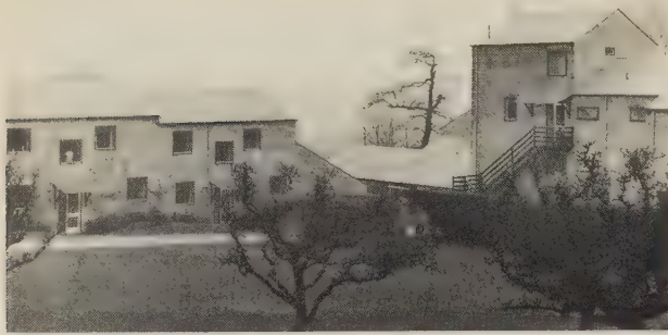
172 MAGUIRE and MURRAY, St John's College Staff Houses , Bramcote, c. 1974. A picturesque version of rural stone architecture done in concrete block. These architects study the vernacular, partly the way Jameson does as a craft tradition, but their emphasis is here in manipulating this as a modest art form. Again the cost and inhabitants' response compare favourably with modernist schemes of a similar size.
