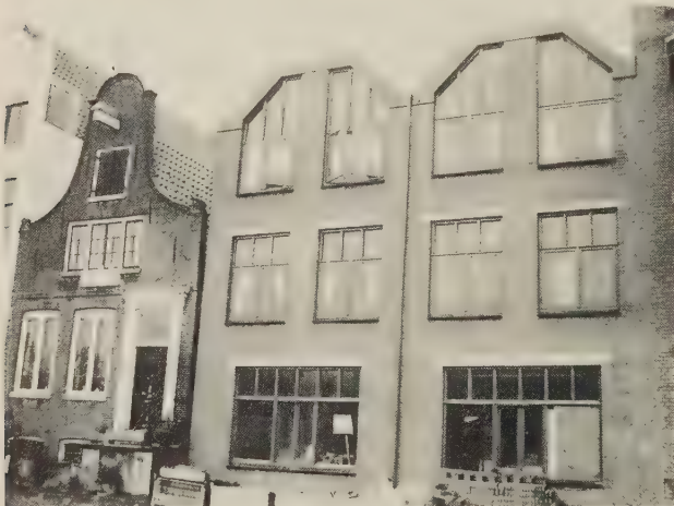
178 VAN DEN BOUT and DE LEY, Bickerseiland Housing , Amsterdam, 1972–6. Narrow, deep houses with oriel windows, 'lightyards' in the centre, truncated gables (compare with the seventeenth century example) and semi-Brutalist detailing. Again a half-way house, or neo -Vernacular job, this cheap housing saved the area from being developed by outside commercial interests, much to the gratitude of the remaining community. An example, like Zwolle , of urban protest resulting in positive action.
