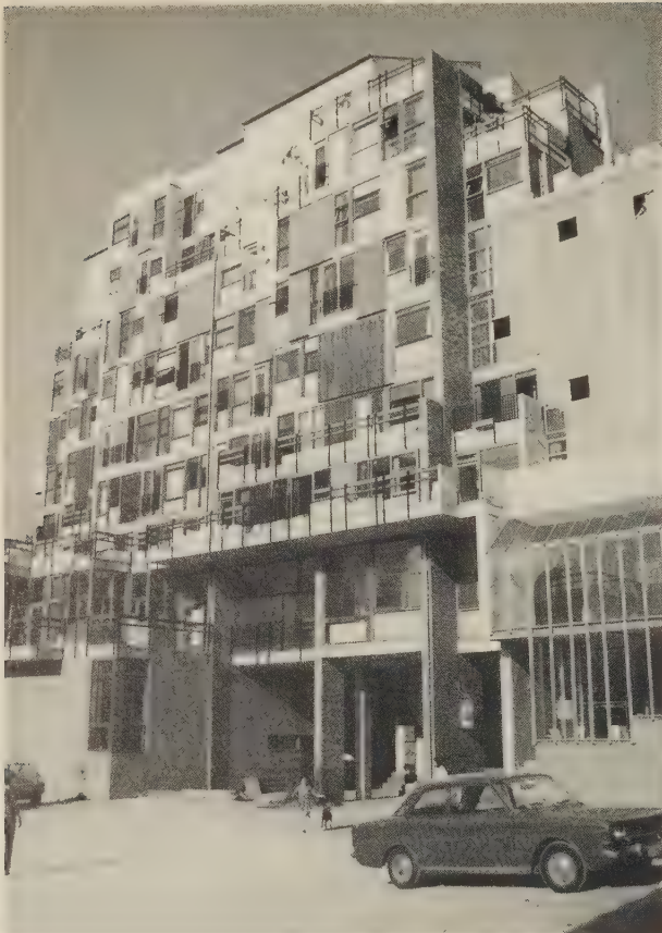
189 LUCIEN KROLL and ATELIER, Medical Faculty Buildings , University of Louvain, near Brussels, 1969–74. An artificial hill town of various activities, articulated with different building systems. The large glazed area is communal, also the restaurant space; the other material – wood, brick, plastic, aluminium and concrete – are also used semantically. Traditional signs are incorporated: greenhouses, pitched roof and chimneys signify the more private areas. The variety and detail simulate the piecemeal decisions which take place over time and give identity to any old city.
