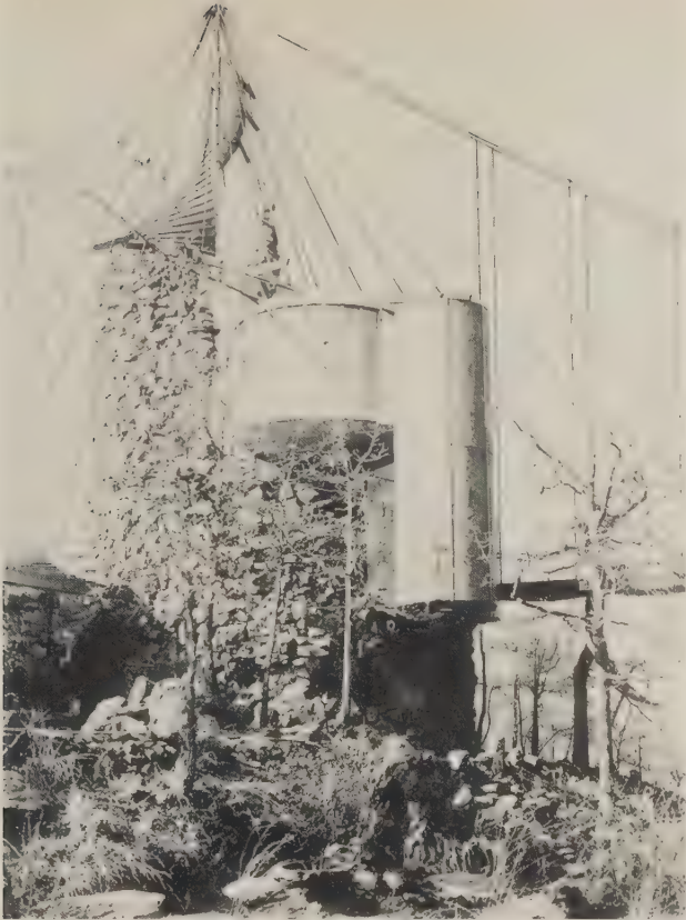
191 BRUCE GOFF, Bavinger House , Norman, Oklahoma, 1957. Goff is the master of ad hoc building, or the 'Army and Navy Surplus Aesthetic', using any conceivable left-over materials. Here a continuous spiral of space is surrounded by sandstone and rubble picked up on the site. A mast and steel cables lifted from boat technology hold up the roof. But he also uses natural, organic materials, such as the untreated, wooden mullions, cut from nearby trees. In addition to all this Goff is the only major architect who uses schlock in a convincing way. He forces us to re-examine taste-cultures which have heretofore been disregarded.
