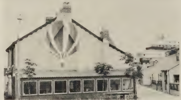
187 RALPH ERSKINE, Byker Architects' Office , Newcastle, 1972–4, in a converted funeral parlour. The red, white and blue graphics rise as optimistically as the balloon on this office in the heart of the renewal. The designers were accessible to the inhabitants who had a say in their future location, neighbours, and type of apartment.
