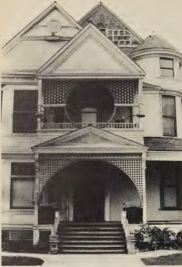
237 J. CATHER NEWSOM, 1330 Carroll Street, Los Angeles, c. 1888. A twelve room house with 'Californian' ornament, lacy spindle and lattice in the 'Moorish manner'. The elaborate shingle patterns, stained glass, circular contrasts and eave recessions add a depth and grandeur to entry. Such virtuosity in wood was helped by the great carpenter-builder tradition which already existed. The results, like Charles Moore's, were not as expensive as they look, and equally wide in reference.
