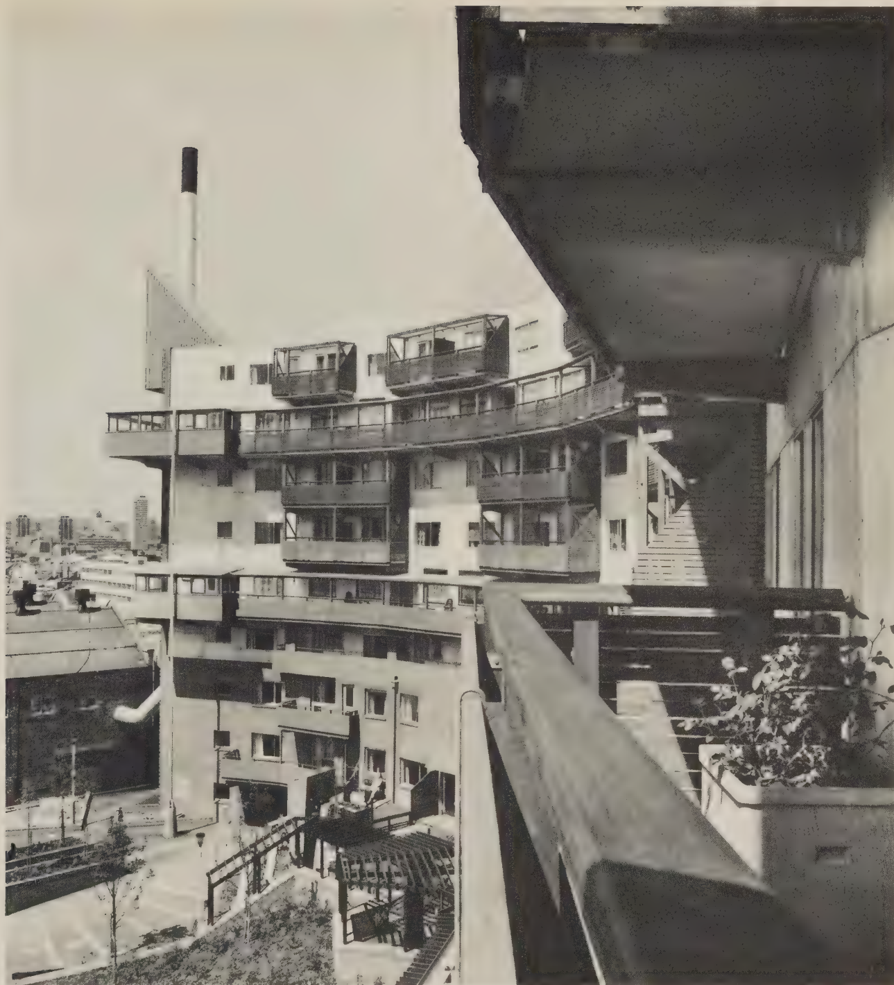
188 RALPH ERSKINE, Byker Wall , Newcastle, 1974. A mixture of materials used in a semantic way: brick in the lower two floors, corrugated metal and asbestos in the upper ones; semi-private deck
