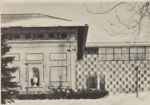
148, 149 VENTURI and RAUCH, Allen Art Museum , Oberlin College, 1973–7. This addition to an Italian Renaissance revival building of 1917 tries to harmonise and contrast with the previous building through its proportions and pink and red stone. Semantically, however, this ‘elegantly decorated shed’ is more a gymnasium than a museum, and awkwardly, not gracefully, integrated with its neighbour.
