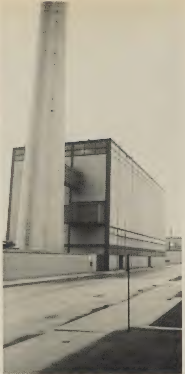
20 MIES VAN DER ROHE, IIT Cathedral/Boiler House, Chicago, 1947 . The traditional form of a basilica with central nave and two side aisles. There are even clerestory lights, a regular bay system and campanile to show that this is the cathedral.
