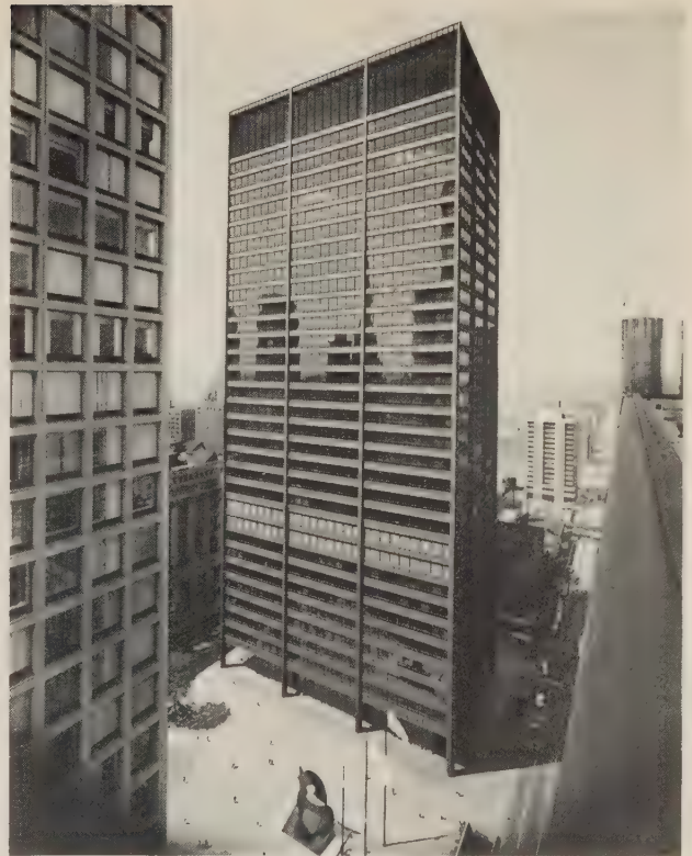
17 C. F. MURPHEY, Chicago Civic Center , 1964. In terms of Mies' curtain wall this solution shows the horizontal emphasis – long spans and underplayed verticals in brown, especially rusted steel. Except for the Picasso sculpture out front, you would not recognise the civic importance of this building, nor the various political functions that occur within. (Hedrich-Blessing).
