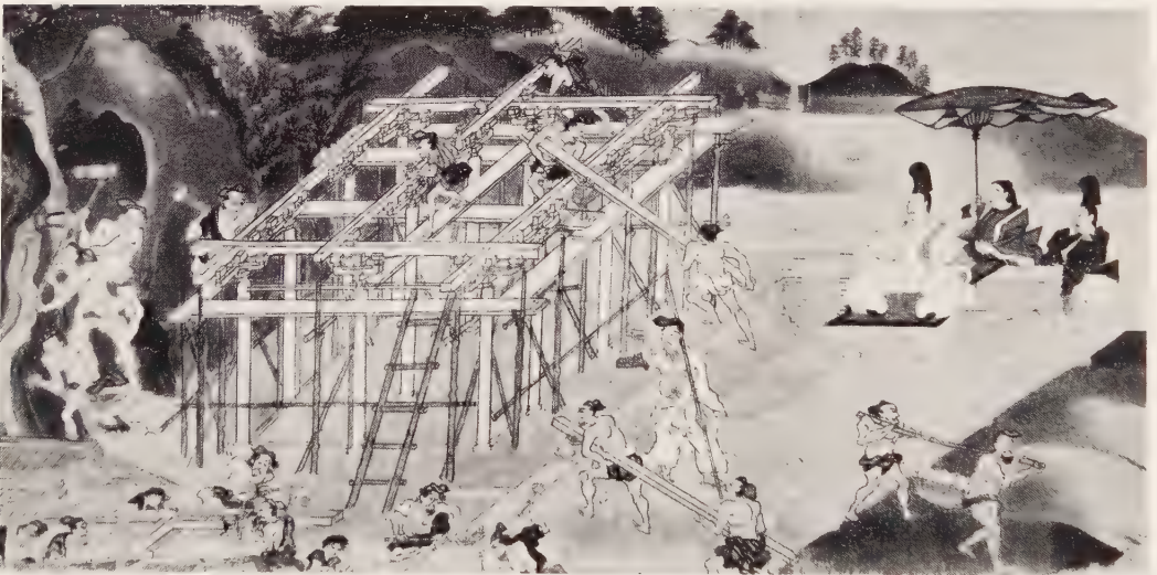
(B) Construction methods, from the Matsuzaki-tenjin-engi
