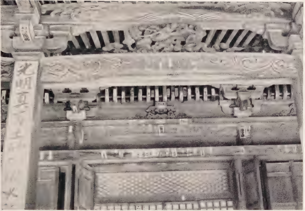
(A) Porch detail. Saidaiji main hall. 18th century
