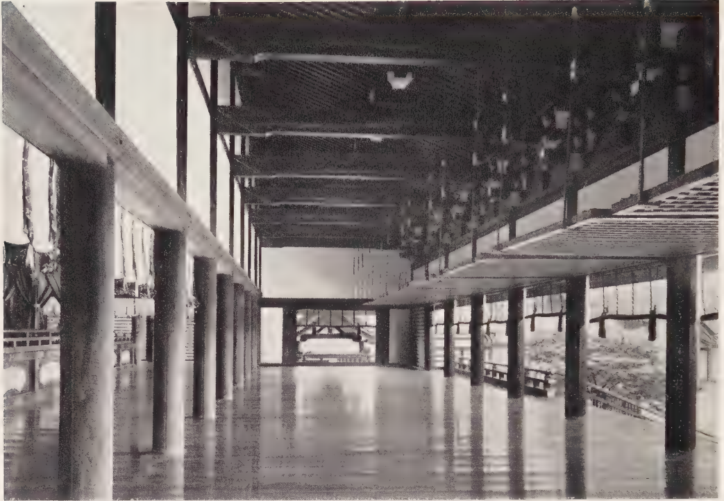
(A) Front veranda, hisashi, of the Shishinden. Imperial palace, Kyōto. 19th-century rebuilding
