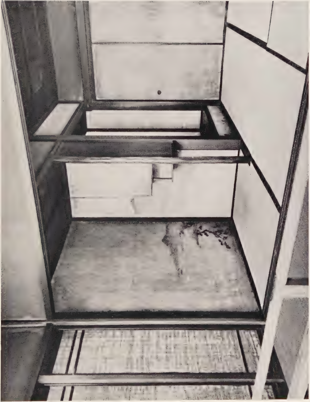
Tea-room of the Ryūkōin of Daitokuji. 17th century
