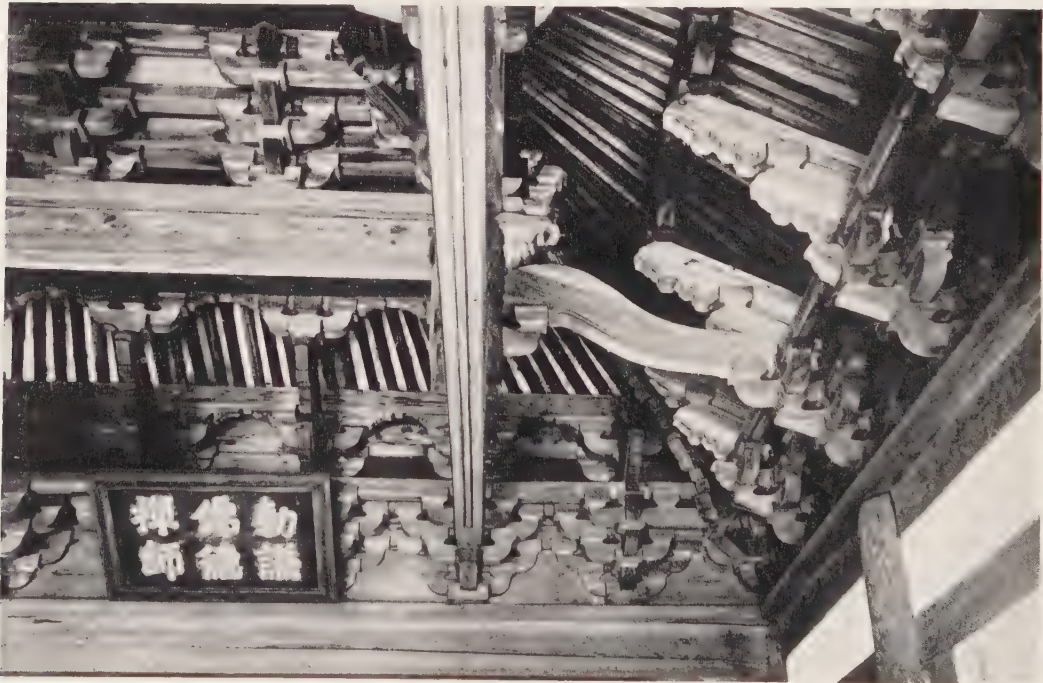
(B) Interior, beam system of fore-hall. Eihōji Kaisandō. 14th century
