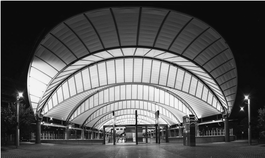
Figure 3.5. Sydney Olympic Park rail station. (© J. W. C. Adam, http://commons.wikimedia.org/wiki/File:Olympicrailstationsydney )
