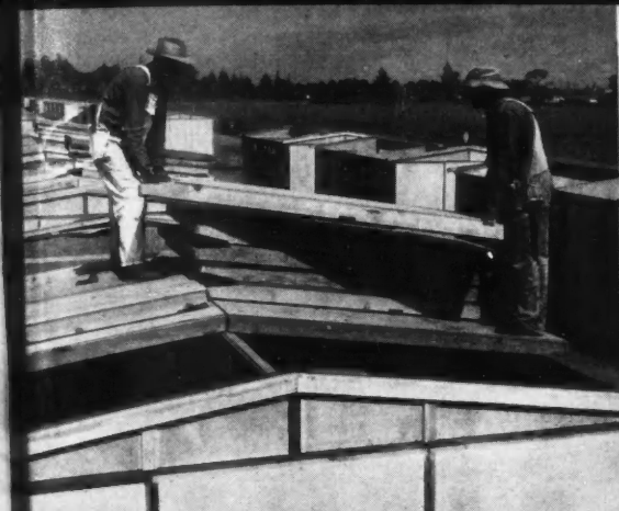
ON GOES THE ROOF
