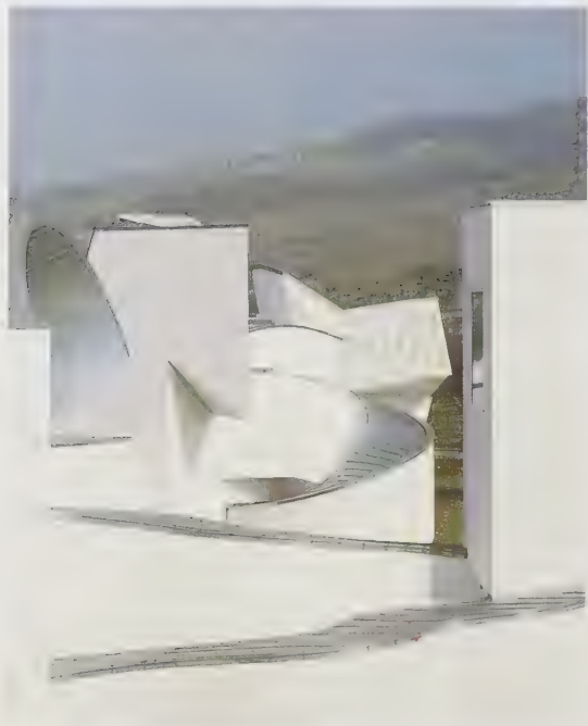
Roofs of the east side of production unit and museum. White plastered walls form a contrast with roofs and wall sections clad in titanium zinc.
