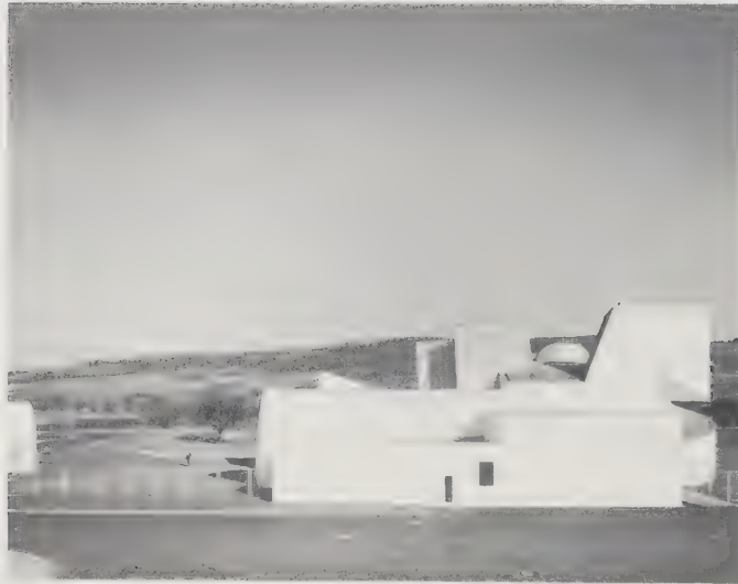
Museum service tract on the factory road. On the right the storeroom with hydraulic ramp, the small entrance on the left leads to office and service rooms. The volumes of this side are designed in such a way as to correspond with the opposite façade of the production unit.
