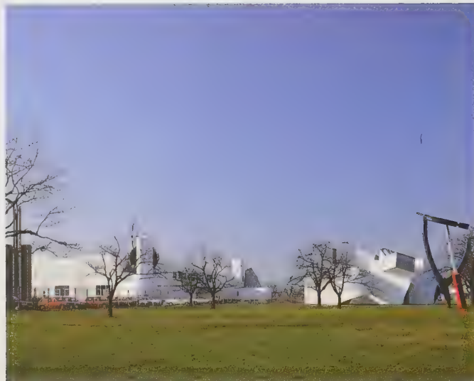
The furniture production unit (left in the picture) with lateral edges emphasized by towers. In the short end of the building opposite the museum are the ground floor production section and loading ramp and upper story with dispatch department. Showroom of Vitra furniture and canteen are reached by side ramps.
