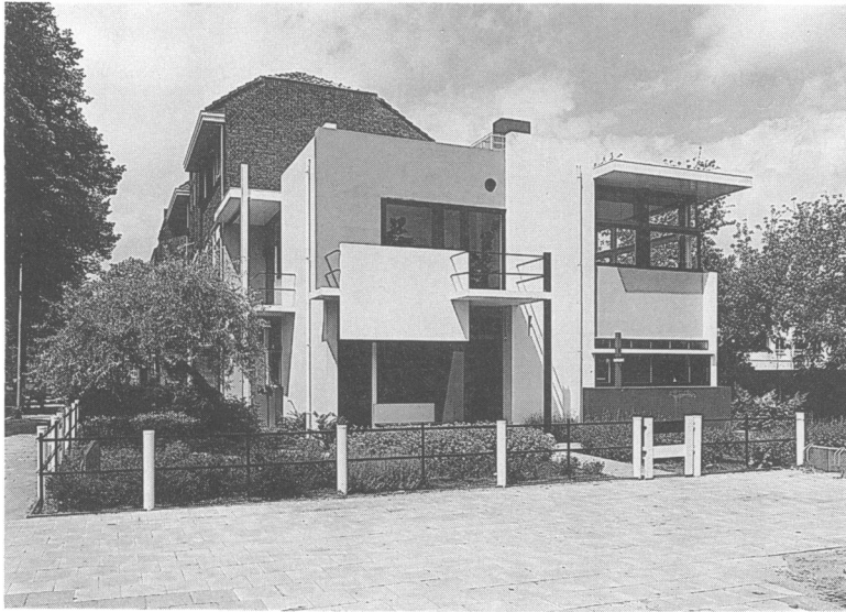
27 Schröder house, designed 1924, exterior; photographed late 1980s
