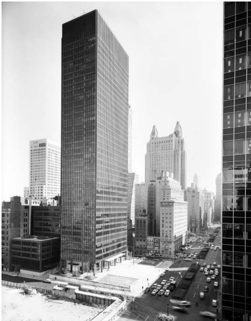
Figure 8 Mies with Johnson, Seagram Building; corner of Lever House, at right, Skidmore Owings & Merrill, Gordon Bunshaft (photo: Ezra Stoller © Esto. All rights reserved)
