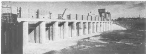
● Iroquois Dam. One of the first large structures nearing completion on the St. Lawrence Seaway Project. On this and comparable projects world wide, contractors continue to prove the best actually costs less with PROTEX.
