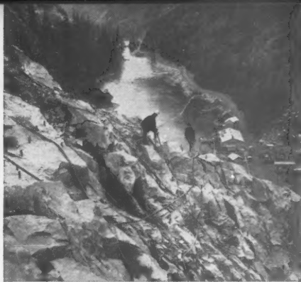
2. Holes are drilled into the overhanging cliff by the drilling crew working for the Merritt-Chapman and Scott Corp., and the Savin Construction Co.
