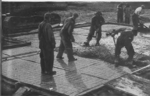
LAI UNDER CONCRETE, Fiberglas-reinforced weatherproof papers put a tough, moisture-proof barrier between the poured slab and the ground.
