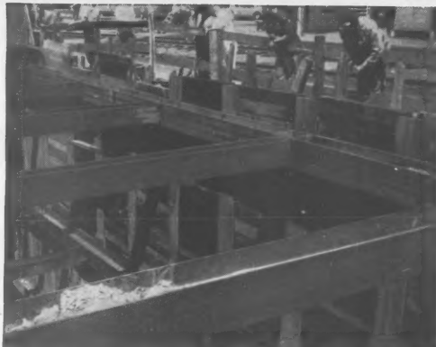
Bethlehem H-piles provide lateral support for excavation for railroad tunnel under construction at Salem, Mass. Contractor: Farina Brothers Co., Inc.
