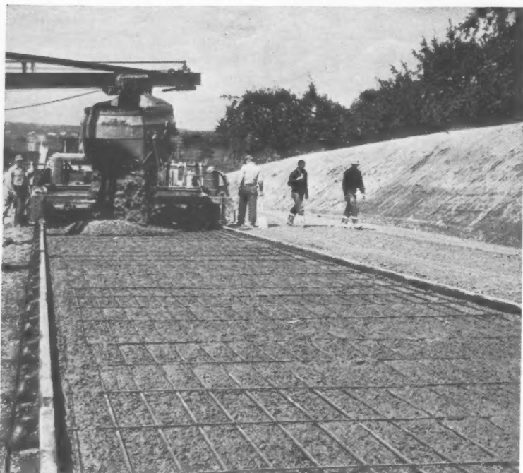
PAVING MACHINE drops a load of concrete for the second 4\frac{1}{2} in. course. About 70 ft of base concrete was laid before the reinforcing mats were placed. The strike-off machine then returned to place the final course of concrete.
