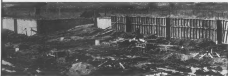
Portion of 300' x 110' poured concrete basement wall 8' to 10' high formed with Rocform Systems for Electrical Products Manufacturing Company, Montreal, Quebec. Entire wall was poured without use of snaptys or wood walers. General Contractor: David Bloom & Company, Montreal, Quebec. Basement Contractor: Rocwall of Quebec, Montreal, Quebec.
