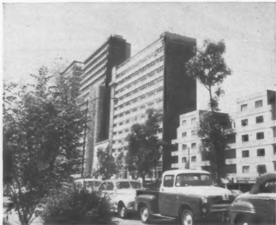
TALL BUILDINGS, TOO , change the skyline. Narrow skyscrapers are popular because they permit day light to penetrate to
