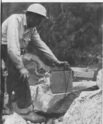
4. The blast is fired with a Du Pont D-48 Blasting Machine, which does away with the need for setting up and maintaining permanent firing lines or blasting generators.
