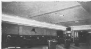
MARINE BANK, Tampa, Fla. —Plaster-Weld applied directly to oil painted ceilings prior to a finish coat of acoustical plaster. ARCHT: Eliot C. Fletcher; GEN'L CONTR: C. A. Fielland, Inc.; PLSTG. CONTR: Joe W. Robertson.
