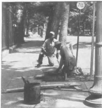
Reduce barricade time and open concrete surfaces for service days sooner by using Columbia Calcium Chloride.
