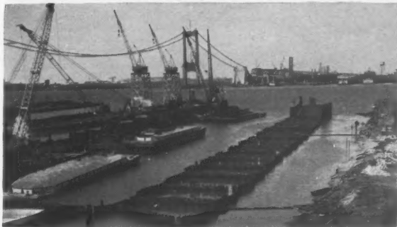
First move was direct placement of coarse aggregate from bottom-dump barges inside cellular sheetpile cofferdam. Barges arrived via Delaware River (rear).
