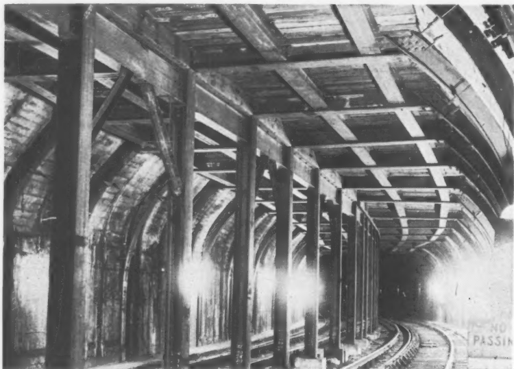
ROOF UNDER A ROOF —Before removing the top of the subway tube, it was necessary to erect a temporary roof within the tube. Setting beams in safety notches added clearance.
