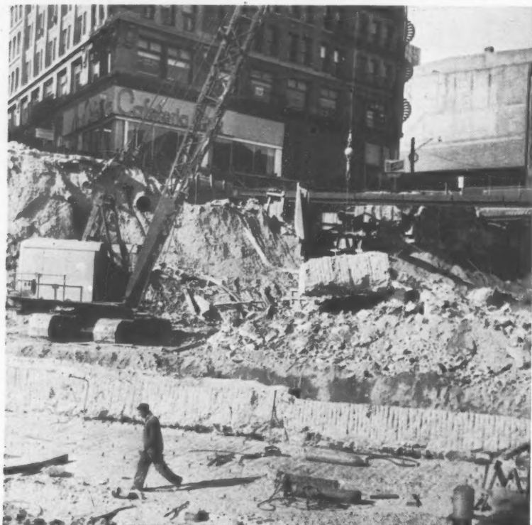
SUBWAY ROOF is of 6000 to 8000 lb concrete with 1\frac{1}{2} in. rods spaced 2\frac{1}{2} to 3 in. on centers, but contractor found a way to remove it in chunks weighing up to 15 tons each.
