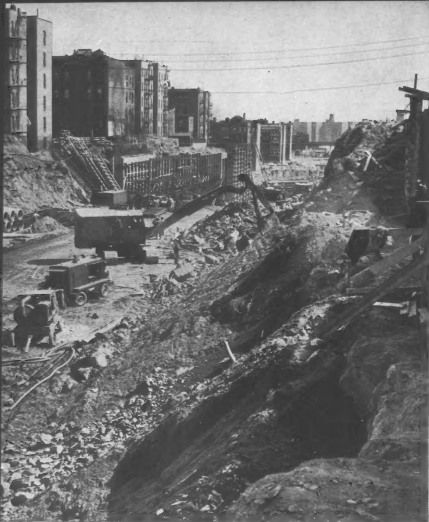
CUTTING THROUGH an area solidly packed with apartment houses and served by a maze of underground utilities is a slow, tough expensive part of adding another link to New York's highway network.
