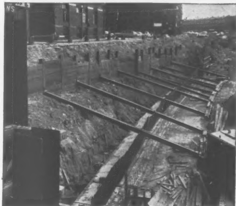
Construction of Boston's Fitzgerald Expressway included placing of Bethlehem H-piles as soldier beams. Contractor: V. Barletta Co.
