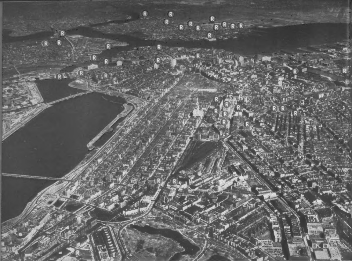
THE RED CIRCLES INDICATE STRUCTURES BUILT ON RAYMOND FOUNDATIONS
