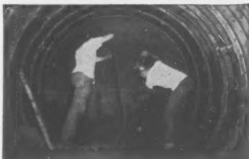
TUNNELING with Armco Liner Plate is quick and safe. Corrugated design features strong overlapping splice.
