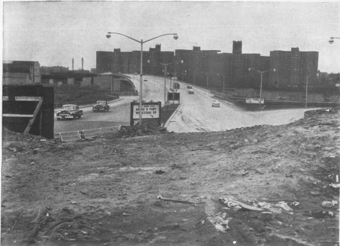
COMPLETED SECTION runs onto construction operations at Longfellow Avenue from which point the Cross Bronx Expressway pushes westward for about 12 blocks to Third Avenue—a distance of 0.8 miles.
