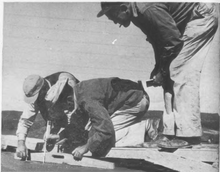
THE NINE INCH SLAB is in place. Department of Highways inspectors check to see that the steel mat has remained at the mid-point of the slab.
