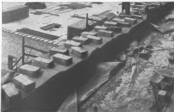
WEIGHTED STRIPS of Fiberglas-reinforced weatherproof papers protect fresh mortar after workmen leave during brick and block construction.
