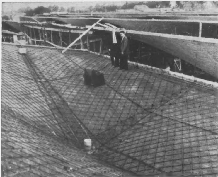
AN UMBRELLA A WEEK is the rate of progress on this factory being built in a new industrial area on the outskirts of Mexico City.
