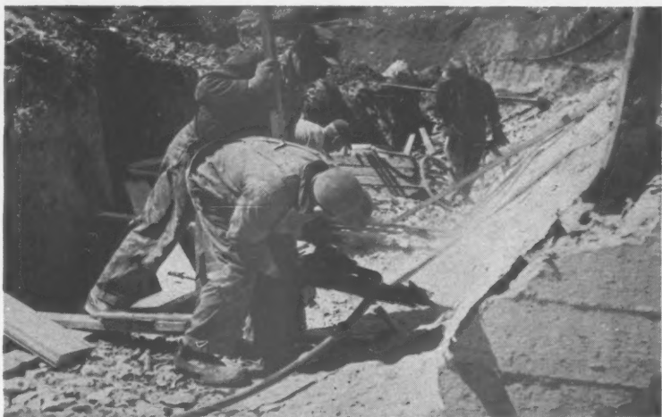
HORIZONTAL LINE DRILLING (foreground) weakened concrete and provided breakage line. Vertical drillers (rear) cleaned concrete from rods for acetylene cutting.
