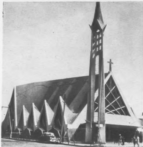
WITH CURVED THIN SHELL CONCRETE SURFACES Architect-Engineer Candela provided the Iglesia de la Virgen Miligrosa with a striking exterior and a roomy interior.
