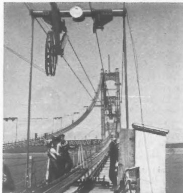
American Bridge Division of U. S. Steel Corporation has strung a total of 12,500 tons of cable as part of the 66,500-ton superstructure.
