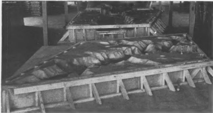
. . . and concreted to form river model sections
