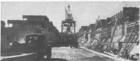
● Grass River Locks. St. Lawrence Seaway Project, Massena, New York. When completed these locks will raise vessels 85 to 90 ft. Projects as this prove the low cost per cubic yard in air entrainment with PROTEX.
