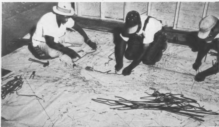
Strap iron is bent to contour lines . . .
