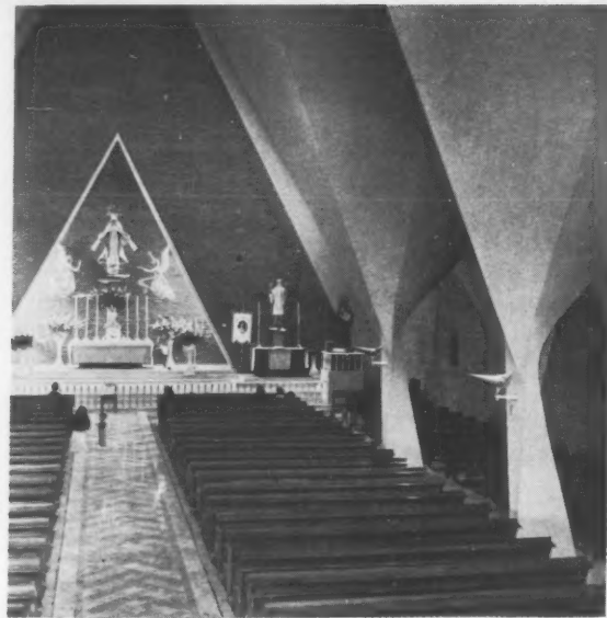
GRACEFULLY SOARING COLUMNS , supporting the thin shell concrete roof of the Iglesia de la Virgen Miligrosa, strike a new note in church architecture.
