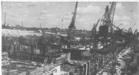
● Massive Barnhart Power Dam. Overall view of power dam construction. This international project being built by the United States and Canada proved the economy of PROTEX.
