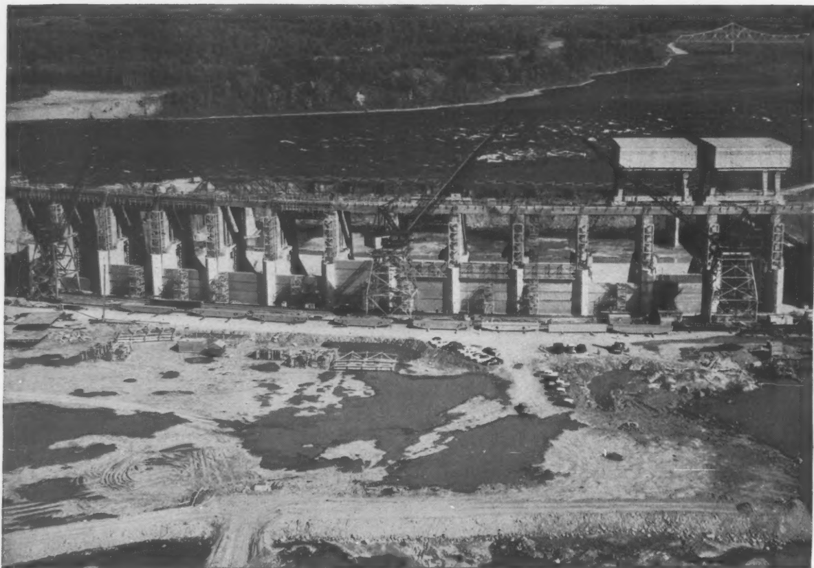
Building the Long Sault Dam. When completed, this dam will contain approximately 653,000 cu. yds. of concrete. The three large gantry cranes used in pouring this concrete are rigged with Tiger Brand Wire Ropes.
