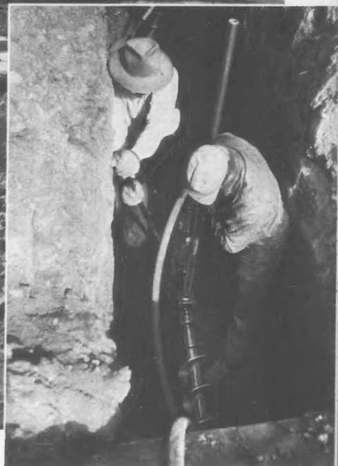
Augering crew preparing to drill beneath the sidewalk for water and sewer lines, using Tractair power.
