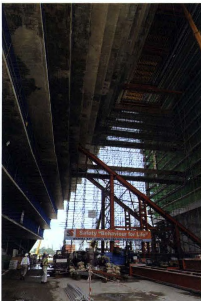
Figure 10. Temporary steel struts for the sloping towers
