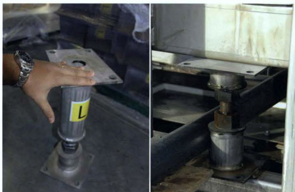
Figure 9. The pool's adjustable steel jacks
