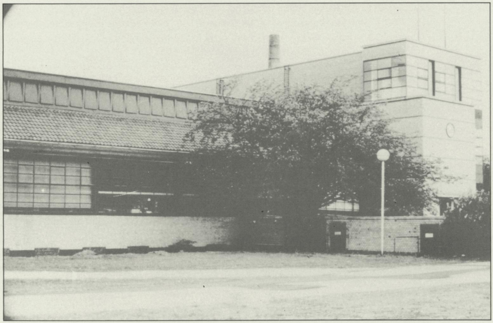
FIGURE 18. View of the Hanover Street front of the Fagus-Werk.
