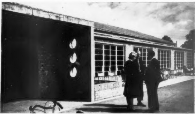
13, INDUSTRIAL HOSTEL, 1941-43, 'composed almost entirely of standard prefabricated huts and units, with a few purpose-built structures to house or emphasize communal activities.'
