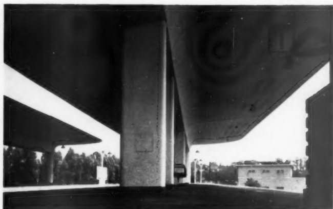
11, SUBURBAN RAILWAY STATION AT LOUGHTON, ESSEX, 1939, with 'its bold sweeps of cantilever and refined detailing . . . [well] in accord with the peculiar functional tradition of [London Passenger Transport Board's] Central Line.'
