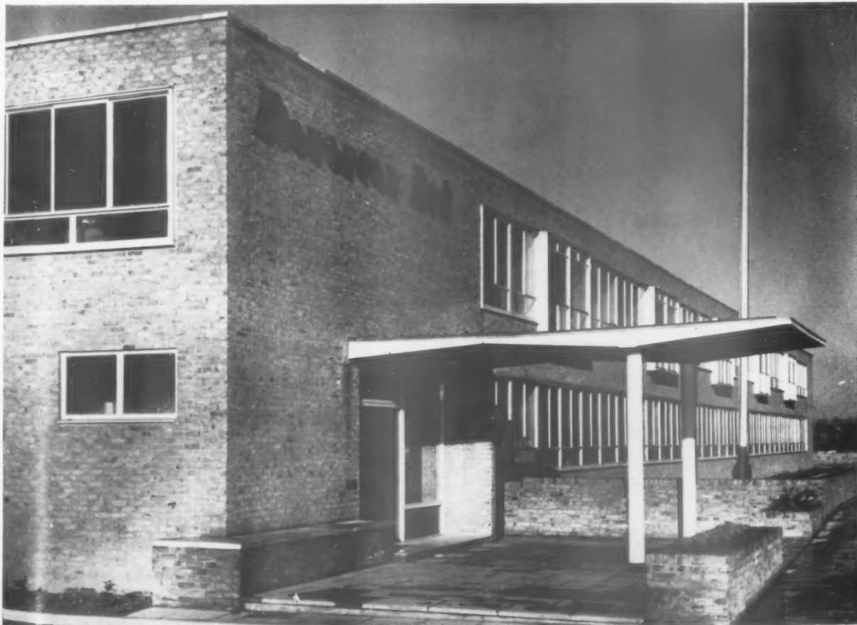
4, the administrative block from the south-east.
