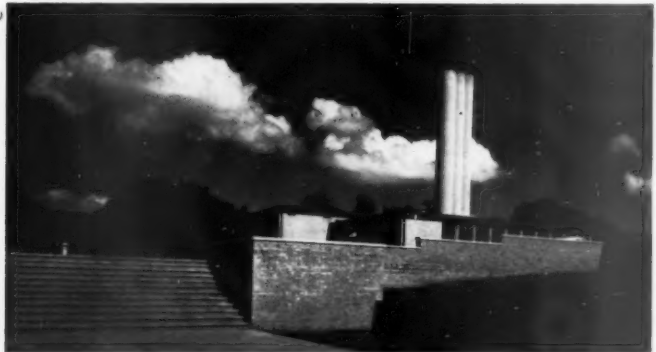
14, BOILER HOUSE AT HATFIELD TECHNICAL COLLEGE, HERTFORDSHIRE, 1952, an 'original and impressive treatment of the [building] and its chimneys as a monumental sculpture on a stepped podium.'
