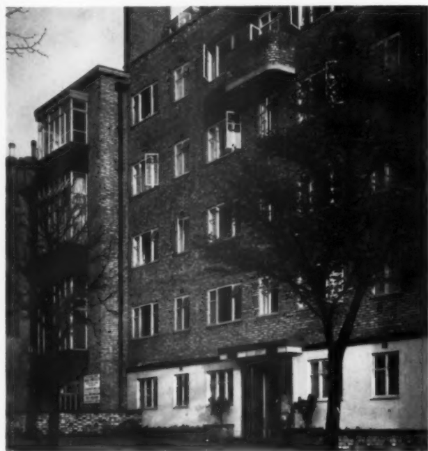
10, ST. EDMUND'S TERRACE FLATS, REGENTS PARK, LONDON, 1938, an ingenious combination of one-and-a-half-storey studio-rooms with the more conventional single-storey flats.
