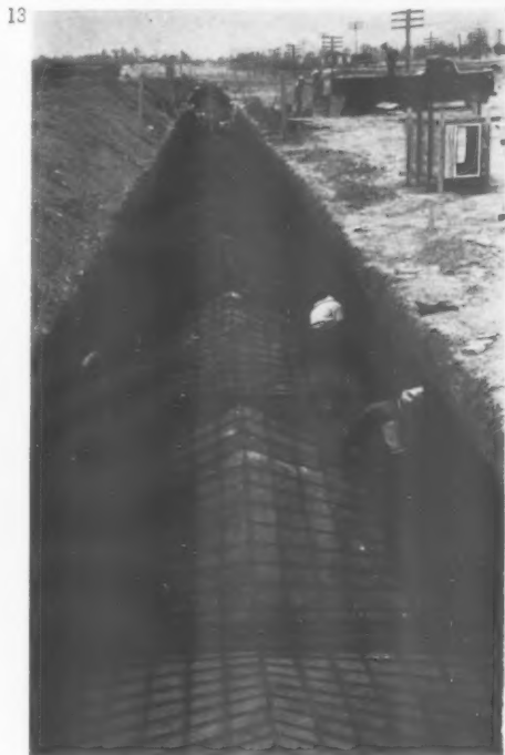
use in inverted form for foundations in 13, while 14 is a mould for making up rein-
