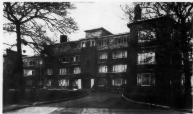
8, AVENUE CLOSE FLATS, REGENTS PARK, LONDON, 1937, a building which in common with the Portman Day Nursery, 4, shows the influence of Robertson's visits to Amsterdam.
