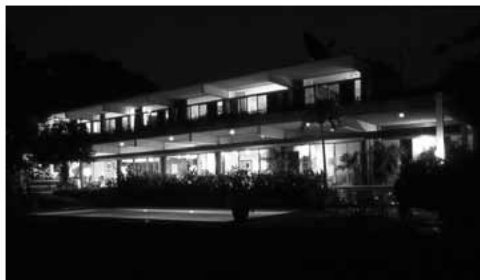
Fig. 11. Richard Neutra , De Schulthess House , Havana, 1956. The transparency of the garden facade suggests a total integration of the building with the tropical garden designed by Brazilian Roberto Burle Marx
